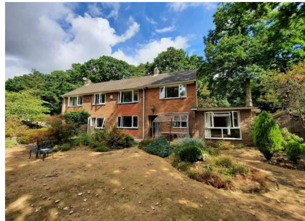
Plate 4.2: Overview of Building 1 Southern Elevation)
