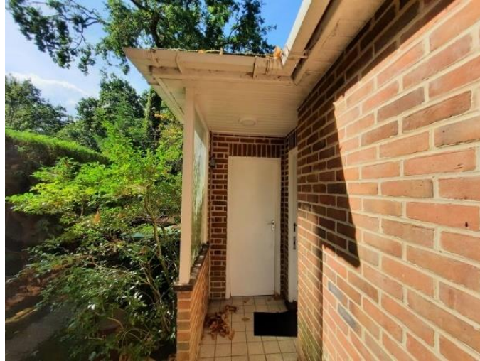
Plate 4.6: Tight Fitting Soffits
