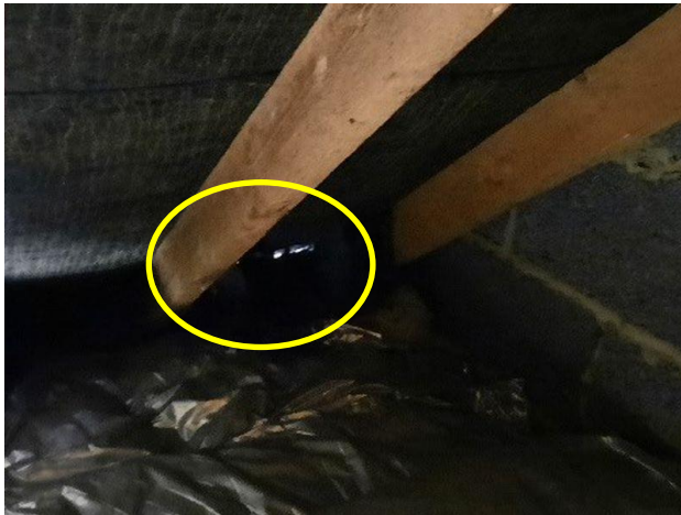
Plate 4.12: Light Entering from Underneath Eaves
