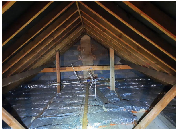
Plate 4.8: View of Ridge Beam
