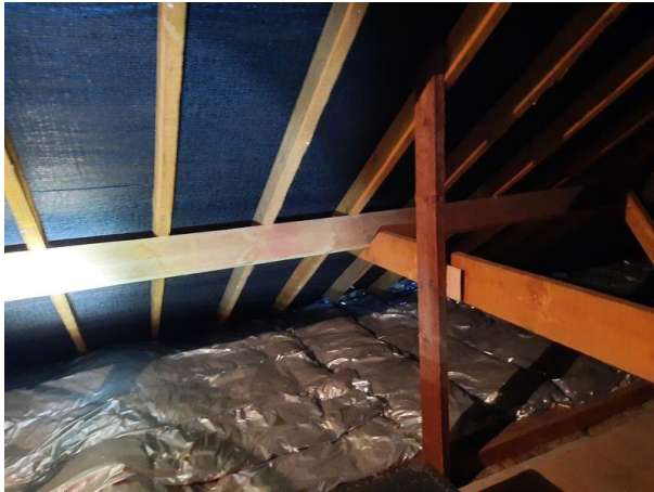
Plate 4.7: View of Felt Sarking
