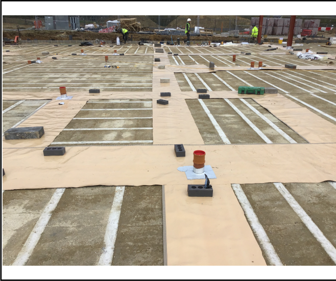
Membrane installation
