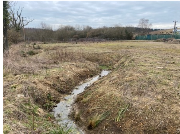
Fig 4. Ditch along northeastern boundary
