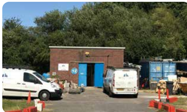
Existing unit 12 to be demolished
