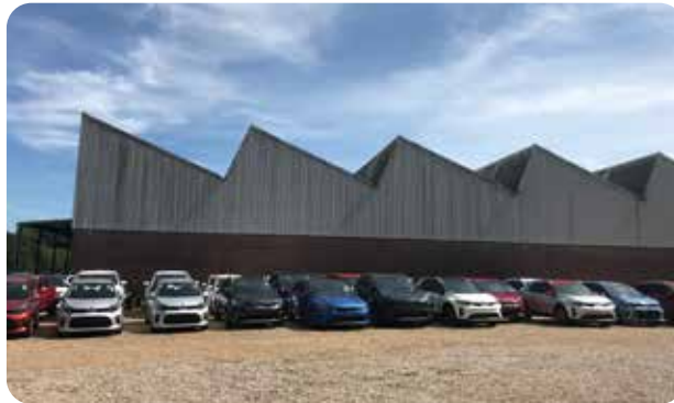
Building 9 South-East elevation
