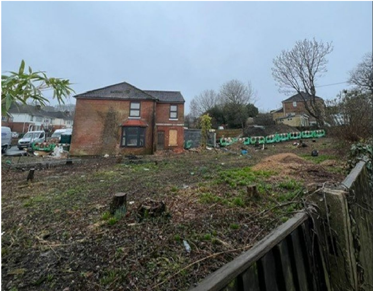
Application site looking south towards No 17 Lower New Road
