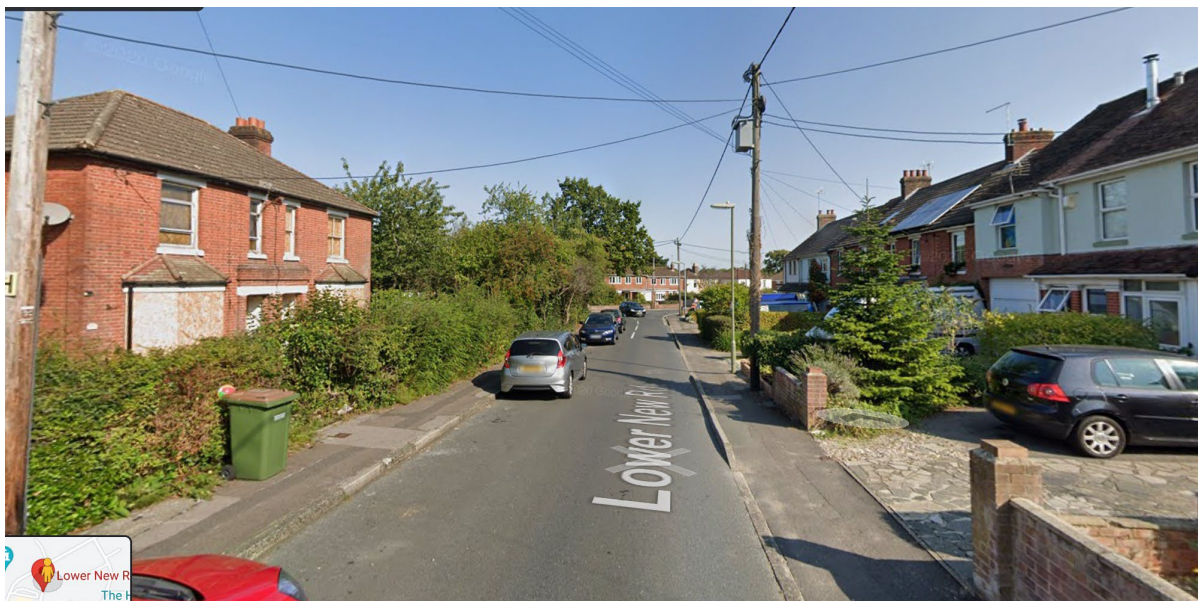
View along Lower New Road looking North ( taken prior to site clearance and works to No 15 and 17)
