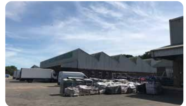
Building 5 in foreground and building 4 in background
