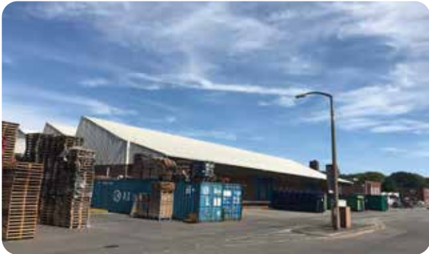
Building 9, view from central estate road
