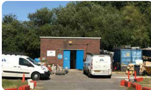
Existing unit 12 to be demolished
