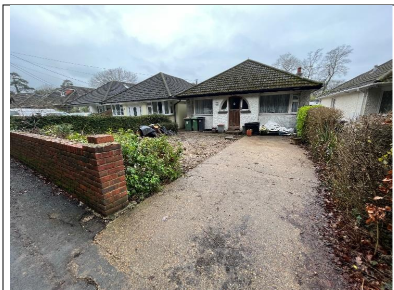
Photograph 1: Building and hardstanding at the site entrance.
