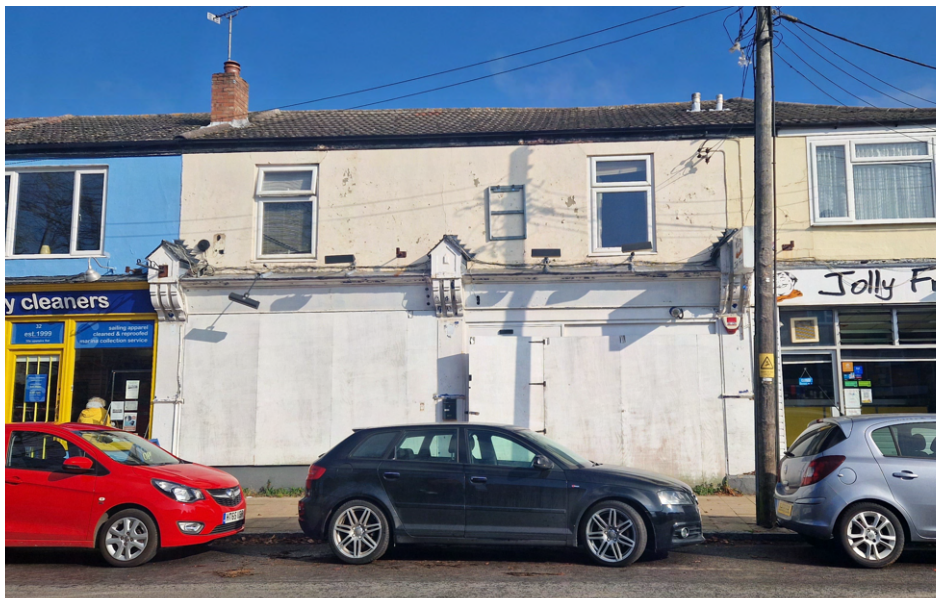
Figure 1: 33-34 Victoria Road, Front Elevation
