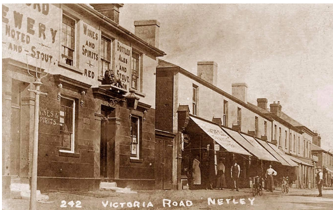
Figure 13: Application Site displaying canopy to frontage
