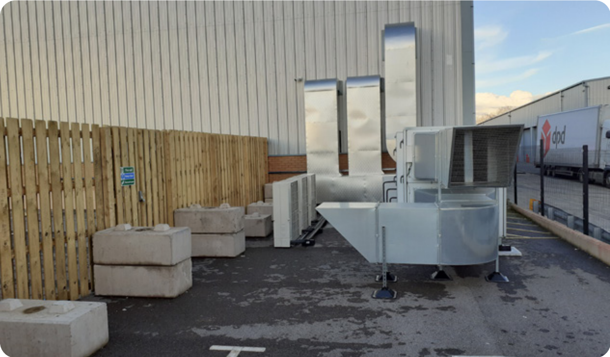
View of the compound looking north east
