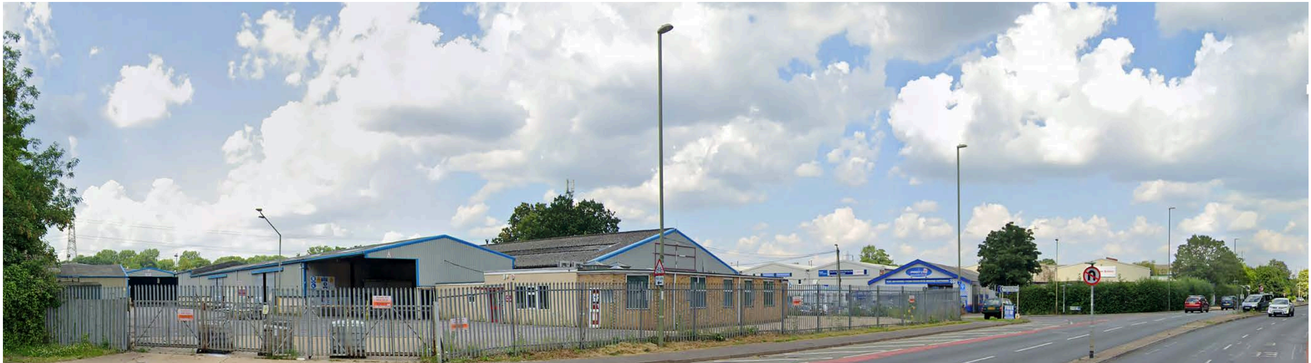
Woodside Avenue - Existing
