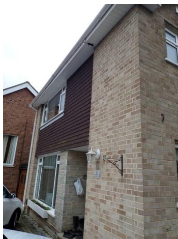
Front elevation with small area of tightly-fitting hanging tiles
