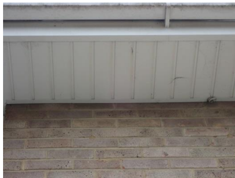
Tightly-fitting uPVC soffits on all sides
