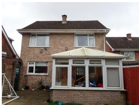
Rear side of house – tightly-fitting Roof tiles, with the odd small gap
