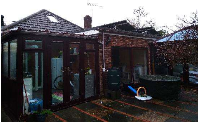
Figure 6: West elevation of the residential building.
