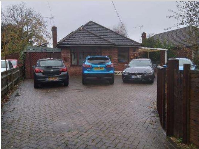
Figure 5: East elevation of the residential building.
