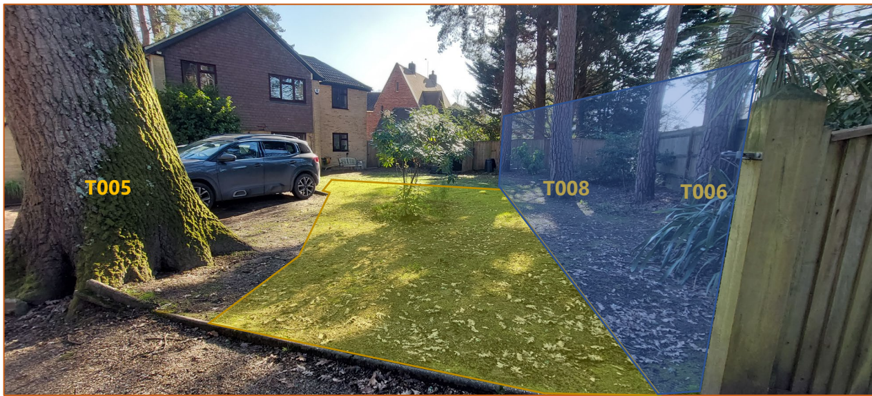
Image 4: The area of yellow annotation illustrates the approximate area of new surfacing required over the RPAs of trees T005, T006 and T008. The blue annotation represents the proposed location of a temporary protective fence.
