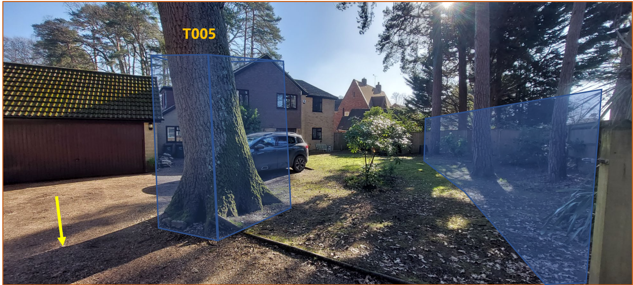
Image 2: The existing surface will be utilised as ground protection and upgraded carefully (yellow arrow). The trunk of T005 and the trees along the front boundary will need to be protected from construction traffic moving in and out of site (as illustrated by blue the annotations)
