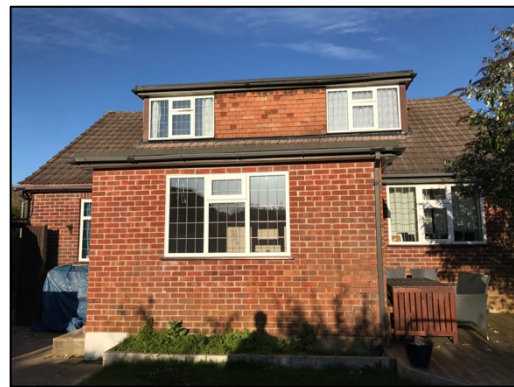
Figure 2 – south-western elevation with extension and dormer windows
