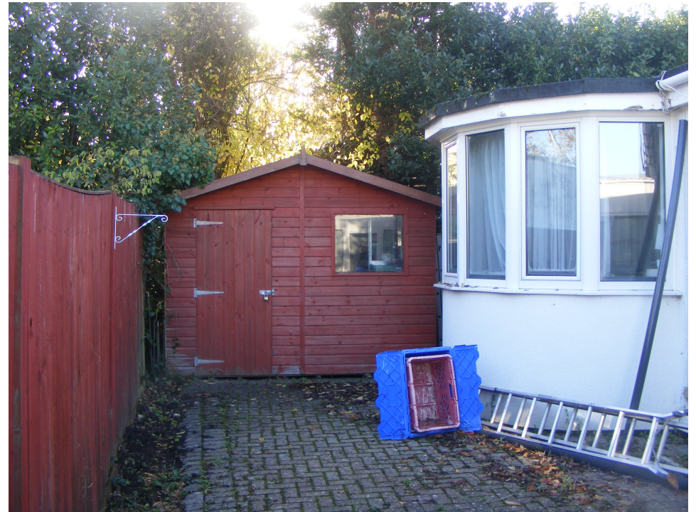
(11) Photo looking South-at the secondary block paved Courtyard Garden Area, adjacent to No.20, highlighting the underused nature of this space, combined with the material quality of the bay window element, due to be completely removed and replaced as part of the property remodelling process.
