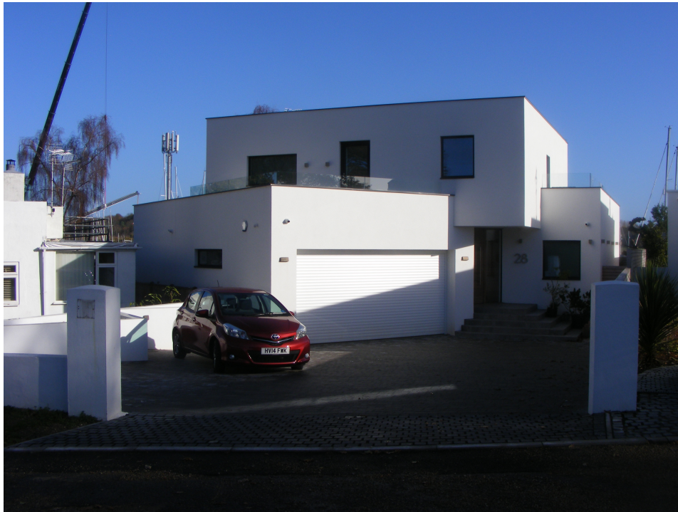
(14) Photo of No.28 Crowsport Estate, a recently extended and remodelled white rendered property with First Floor and Roof Terrace accommodation, as per Planning Approval C17/80337 (details confirmed in Appendix A).
