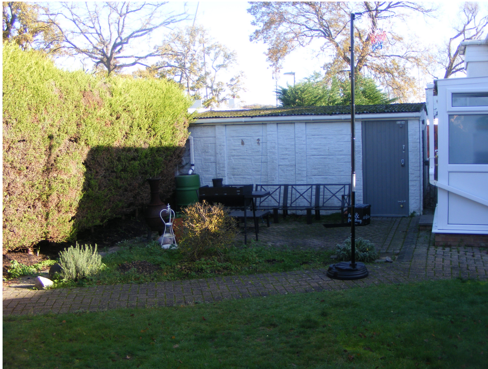
(08) Photo looking East from within the front “Courtyard Style Garden” at the side of the existing Double Garage, due to be demolished and reincorporated into the volume of the remodelled dwelling.
