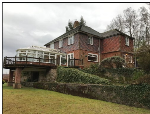
Figure 7 – north-eastern conservatory and balcony
