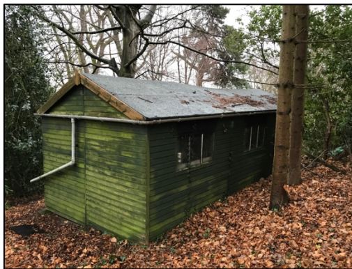
Figure 12 – wooden built shed outbuilding
