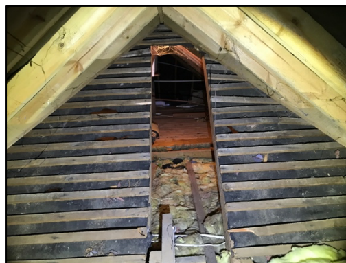
Figure 9 – roof void entrance to hipped extension
