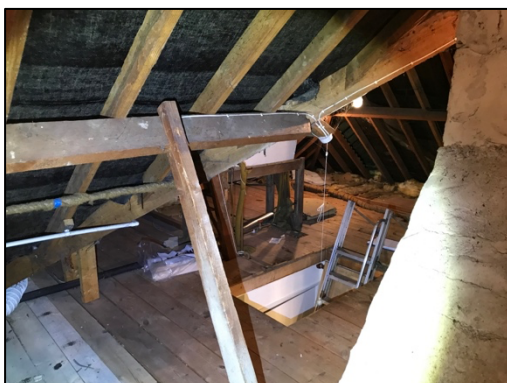
Figure 8 – roof void of main house with central chimney
