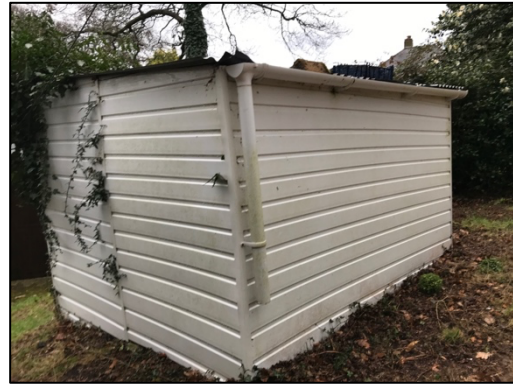
Figure 15 – northern and western elevations of the outbuilding
