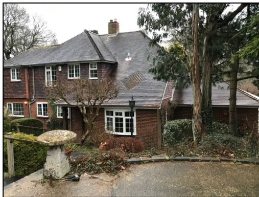
Figure 5 – south-western elevation with catslide roof
