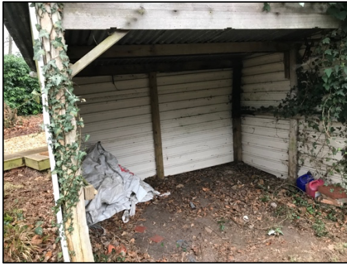
Figure 14 – open eastern elevation of outbuilding
