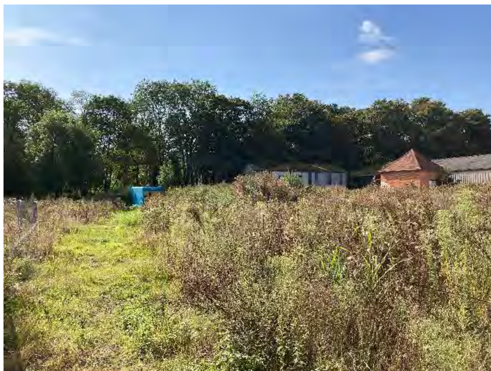
Photograph 6: View of Stockpile 3 (SP3) and the western part of the site, looking west.
