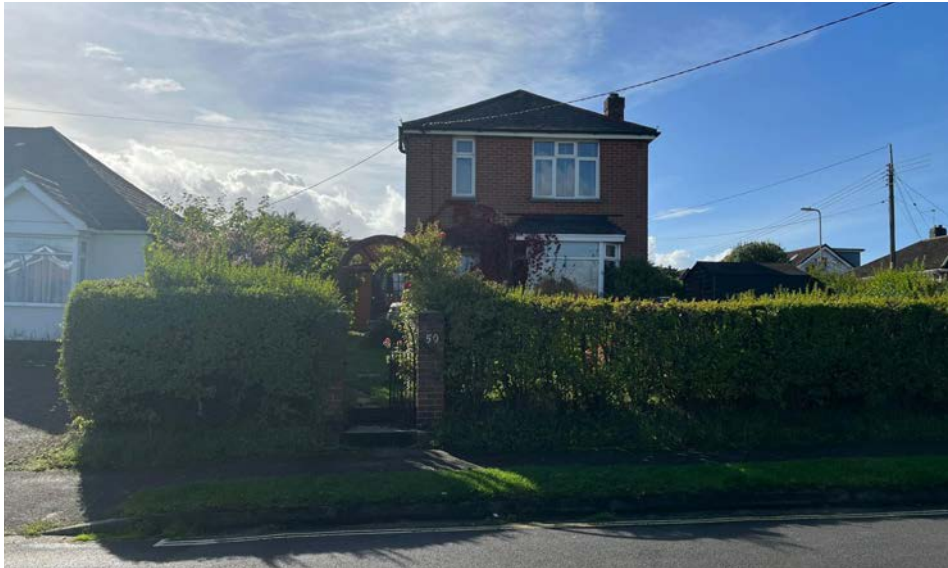
Site photo from Sharftesbury Avenue
