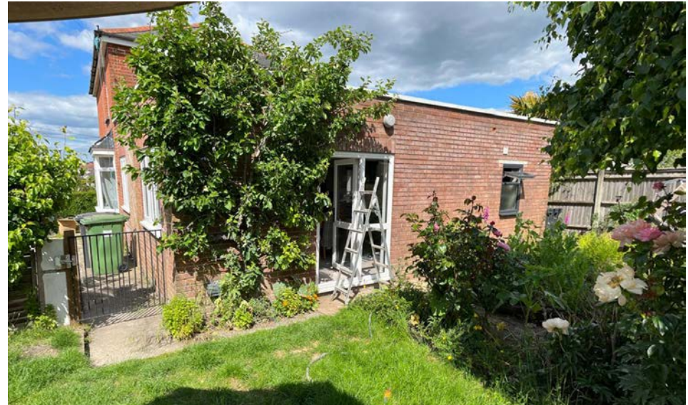
Site photo from the rear garden
