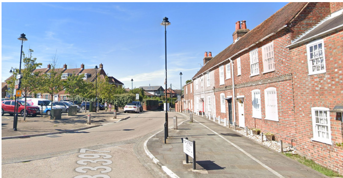
Figure 12: View from Copperhill Terrace (Closest Listed Buildings)
