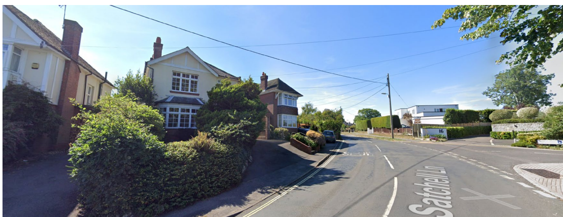
Figure 4: View from highway looking towards Crowspoint, modern flat roof developments (within the conservation area)
