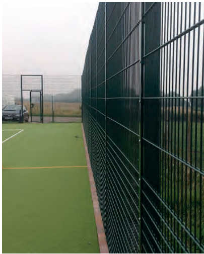
AGP single leaf (pedestrian) and double leaf (maintenance access) gates to match adjacent fence
