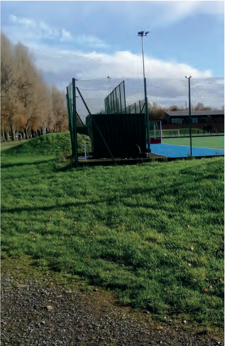
Existing aggregate paths in proximity to the existing artificial pitches
