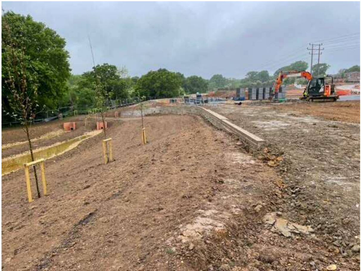
Photograph 5 : pond looking, tree planting to banks installed, upper wall also installed to serve perimeter footpath
