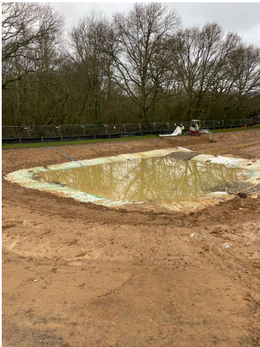
Photograph 1 : pond stilling upper basin installation, view south west
