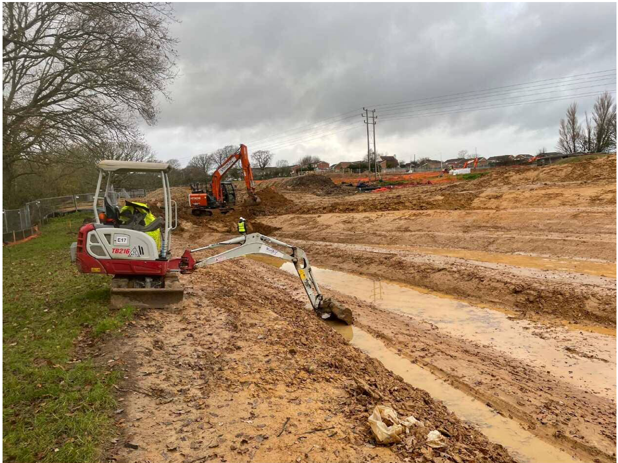
Photograph 4 : Excavation of the pond channel system, view west
