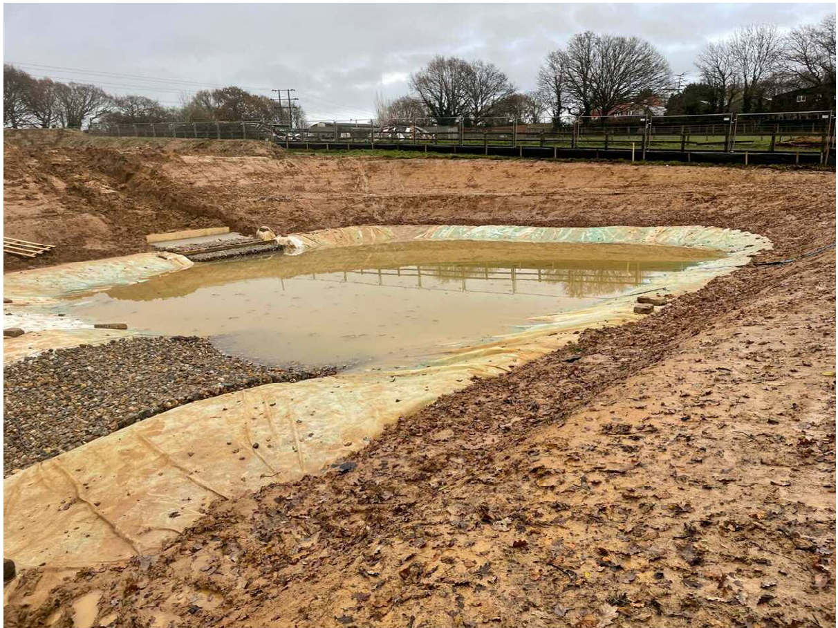
Photograph 2 : Pond looking north east, outfall matting visible as in the liner within the geotextile
