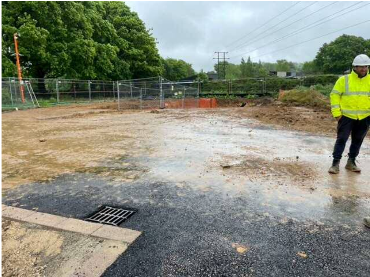
Photograph 2, Macadam surface over porous paving
