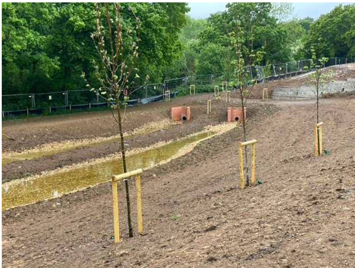
Photograph 4 : pond looking south west, tree planting to banks installed, masonry headwalls to channel system visible
