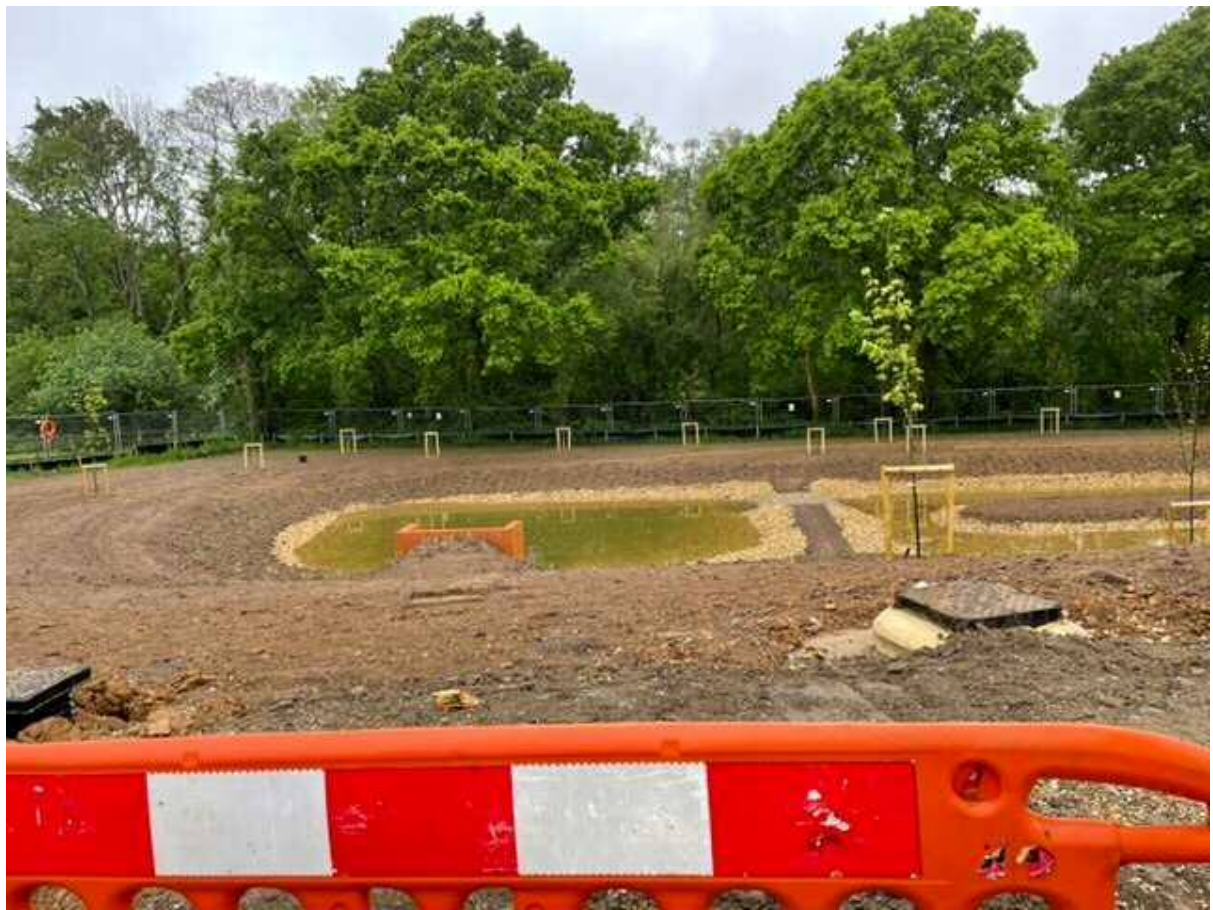
Photograph 3: pond looking south, finished masonry outfall and mattress visible
