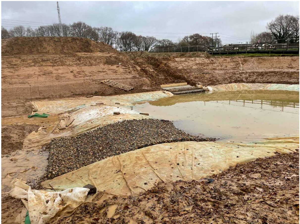
Photograph 3 : Pond looking north, transition weir to foreground
