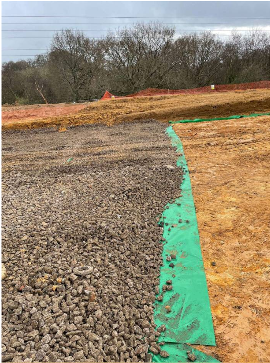
Photograph 4 : Early installation of the porous paving, liner and 'no fines' stone material recorded
