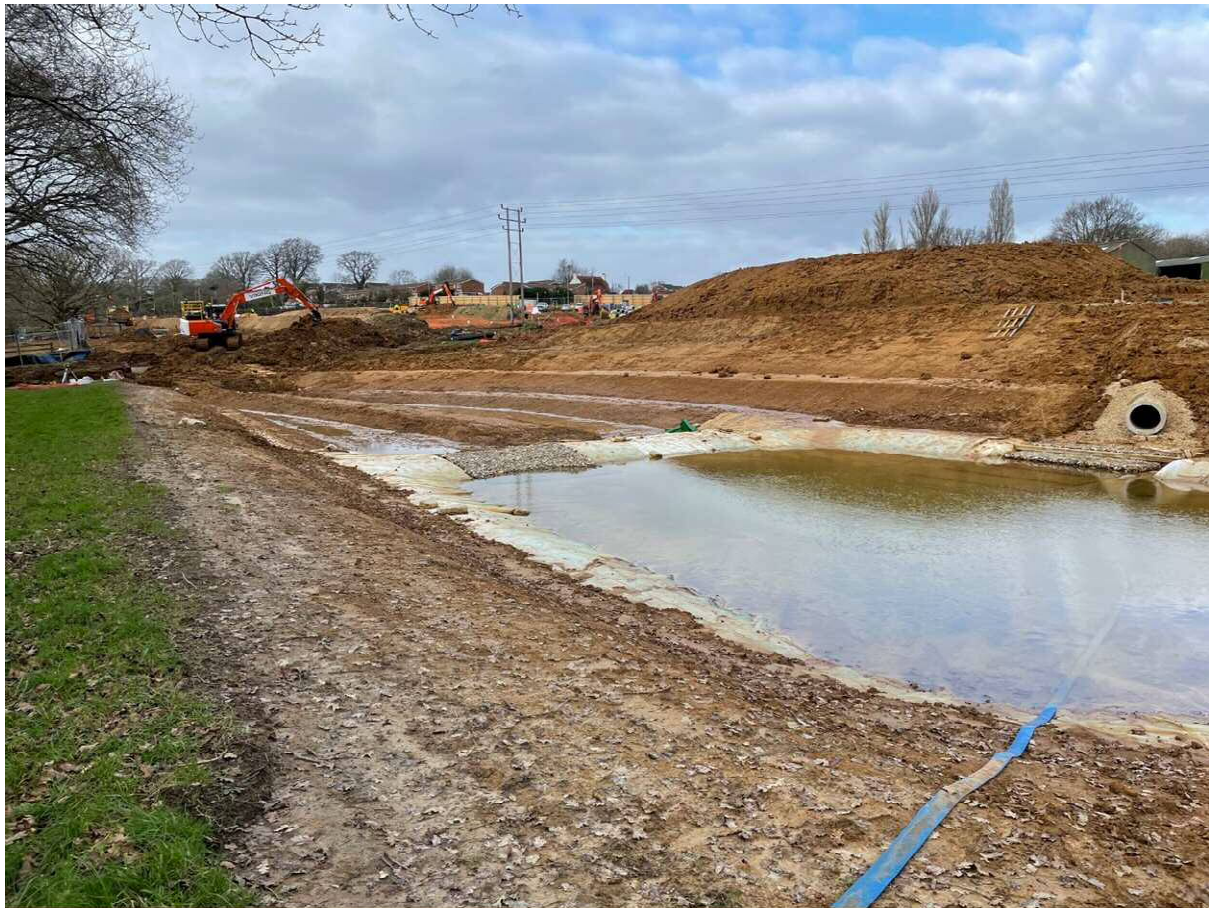
Photograph 3: pond looking north, outfall and pond liner visible
