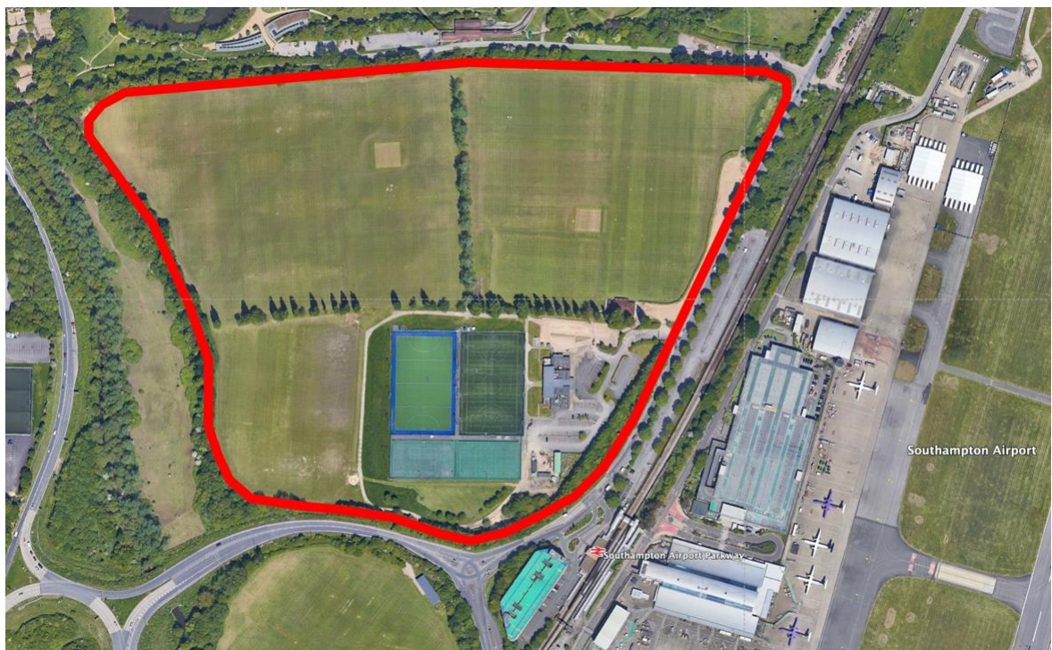
Figure 1. Wide Lane Sports Ground
