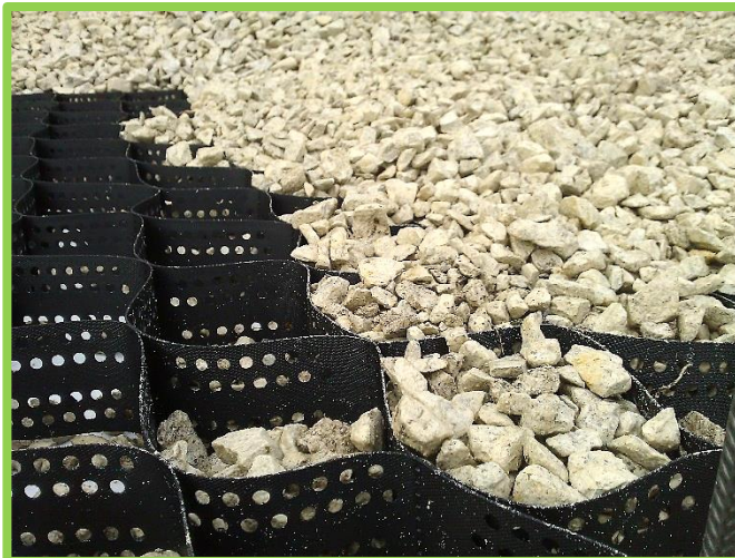
Arboricultural Protection Method 2 – Temporary Ground Protection
