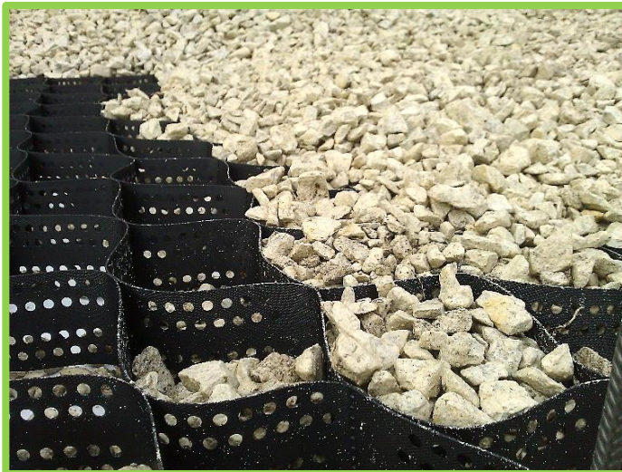
Arboricultural Protection Method 7 - Installing Hard Surfacing - Tree Root Protection within RPAs
