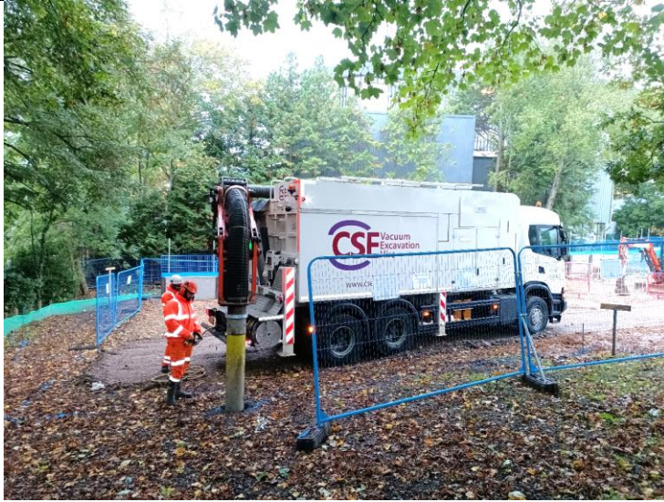
Vacuum Excavation for a Lighting Column within the RPA of retained trees
