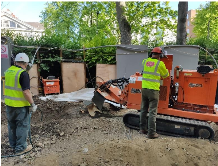
Excavation by grinding machine of stumps within the RPA of retained trees by tracked grinder under supervision from an arboriculturist.
