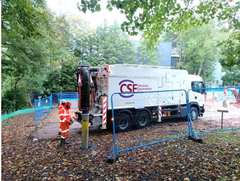
Vacuum excavation for a new Lighting column within the RPA of offsite retained trees.
