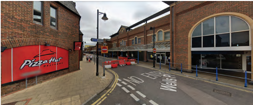
1. Looking East Along Wells Place
