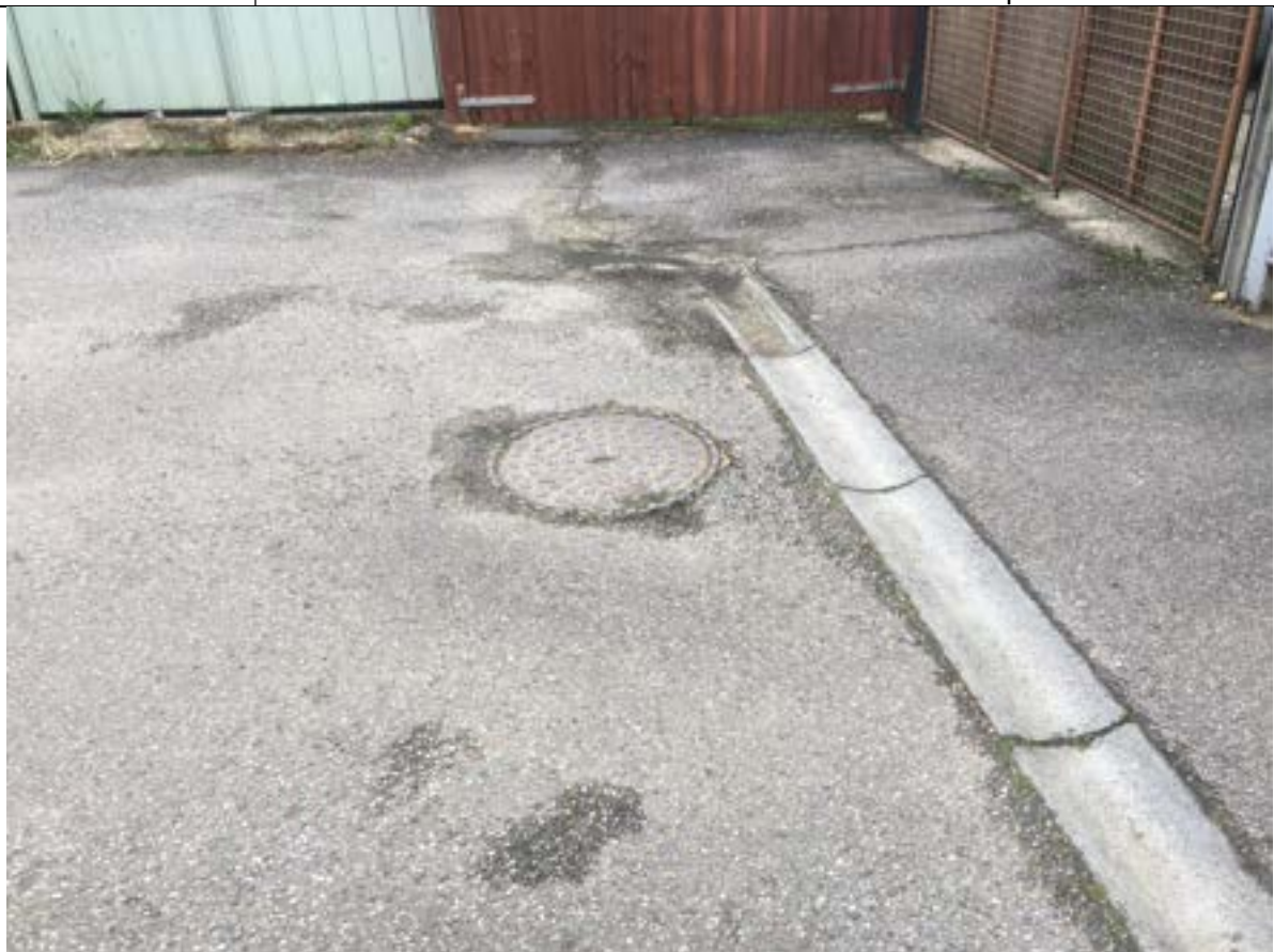
Photo 6: View from Northeast site corner of off-site Mains and Surface Drainage
