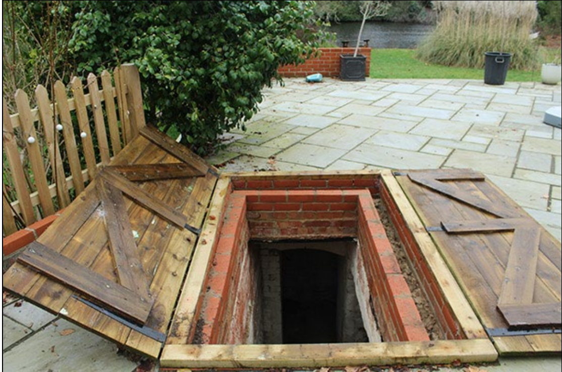
Figure 8 The wooden hatch leading down into the cellars of The Hermitage
