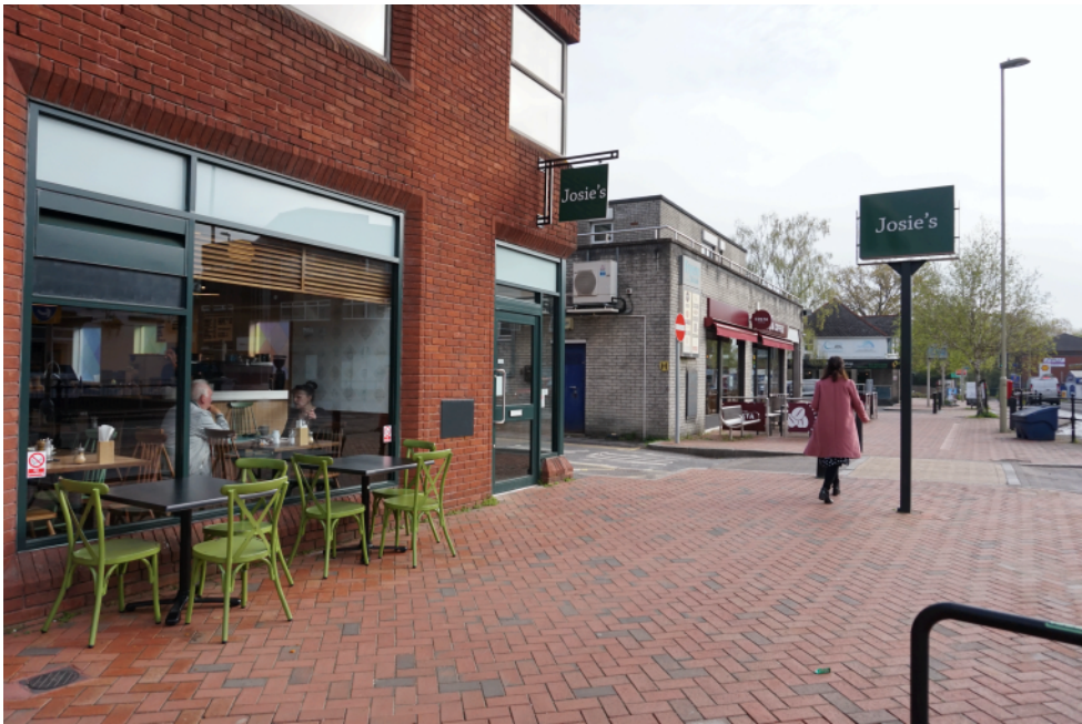
Josie's - Applicant's Site Exterior Photograph - As Built (Retractable Awning Yet To Be Installed)
