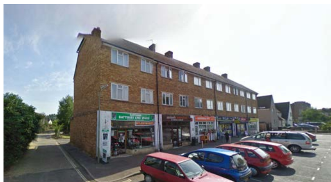
Nightingale Avenue Retail Parade- with access to side towards site.
