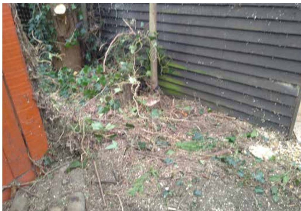
Looking south-west, showing the removal of the trees
