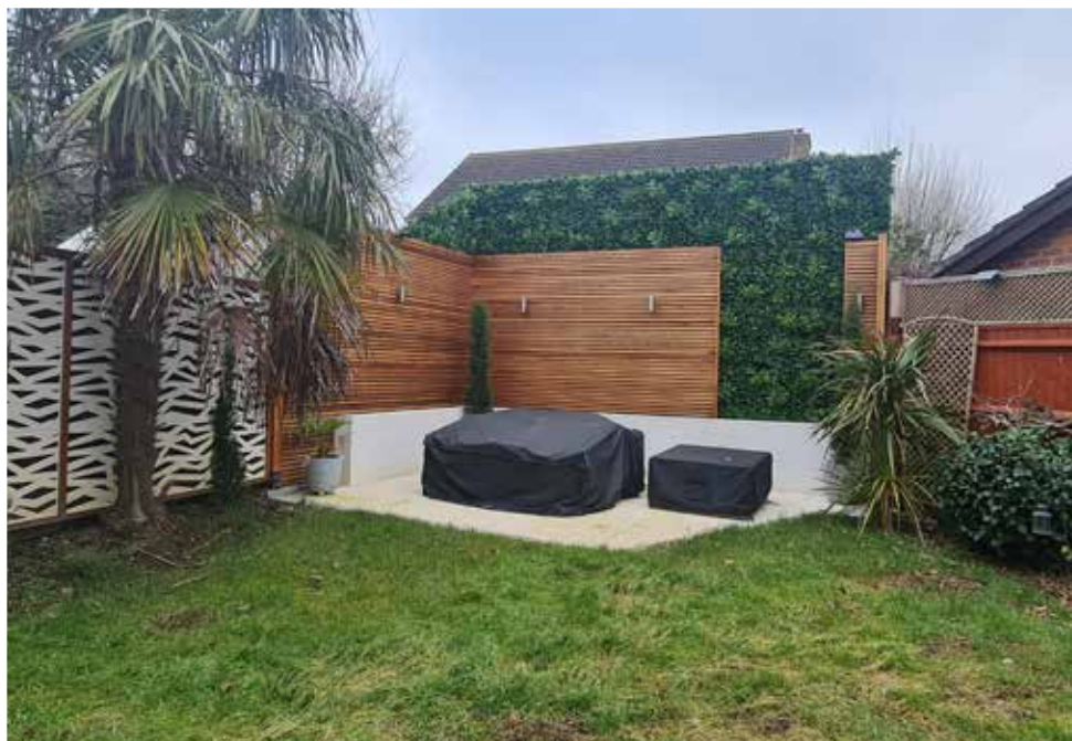
The completed works at No.6 Luxton Close (taken February 2023), with following implemented: - Timber slat cladding to mimic the stepped fencing at the boundary with No.7 (from top of white wall up to normal fence height) - Upper area of acoustic fence clad with greenery to mimic the former line of trees (at a reduced height)
