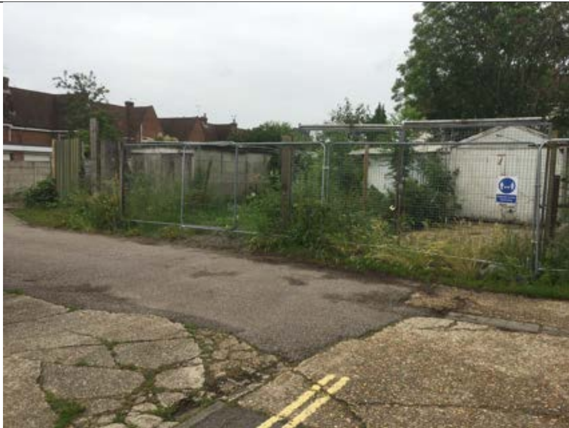
Photo 1: View Southwest of Garages
