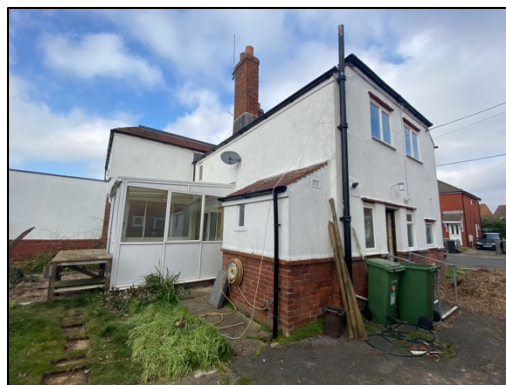
Figure 2 – rear conservatory and brick-built extension
