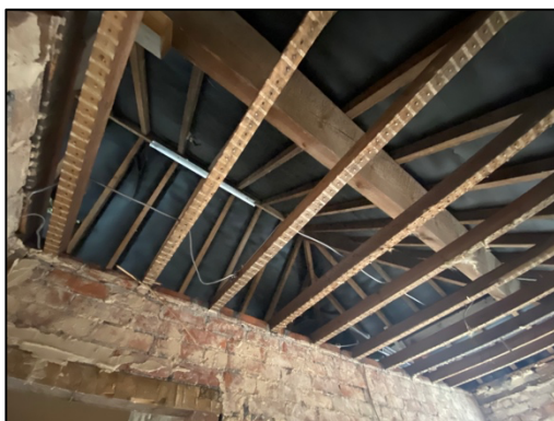
Figure 3 – open interior with exposed bitumen lining
