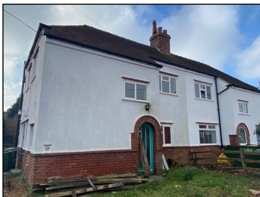
Figure 1 – north-eastern elevation of the house
