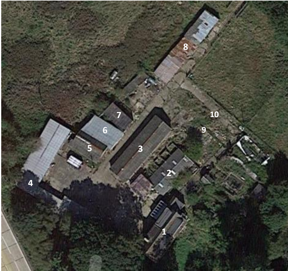
Figure 15. One dwelling and 9 outbuildings on site with their associated numbers.
