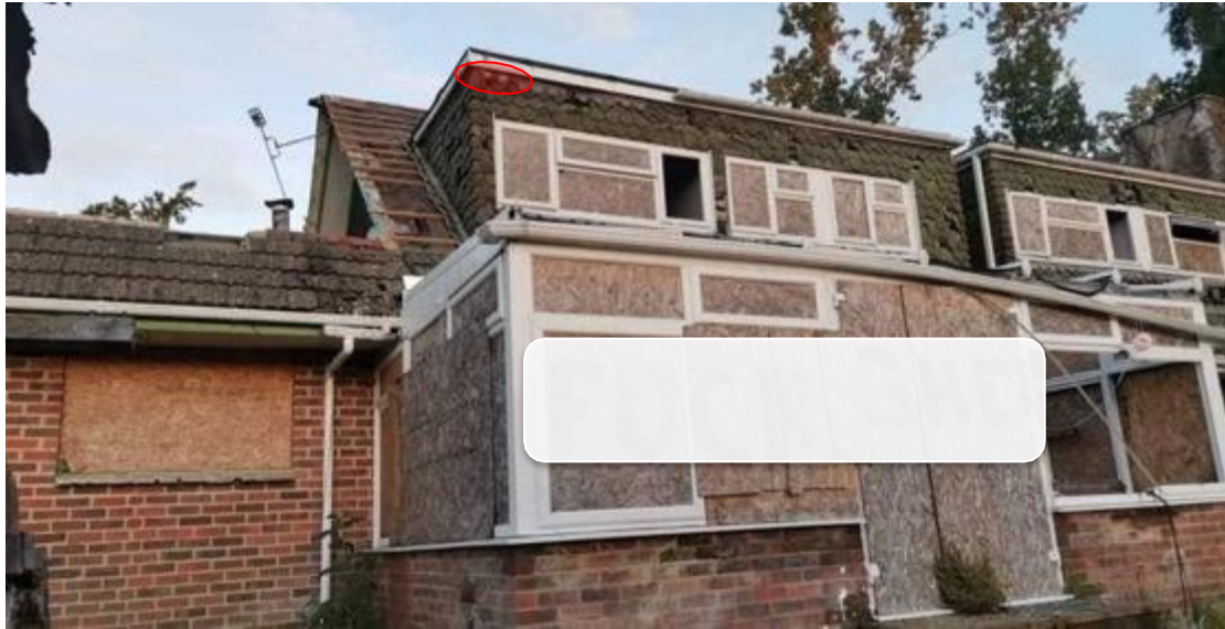
Figure 28. Approximate locations of 2 x Common Pipistrelle emergence (Red dot) on the north west facing aspect during the first survey.
