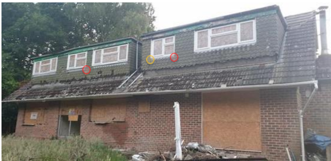
Figure 29. Approximate locations of individual Common Pipistrelle emergences (Red dot) and 4 Common Pipistrelle and 1 Soprano Pipistrelle (orange dot) on the south east facing aspect of the dwelling.
