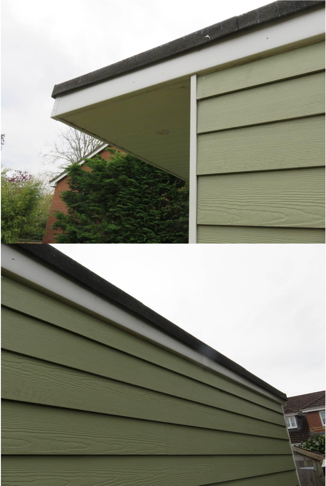
Photo 12/13 Felt Roof and cladding construction, No evidence recorded.
