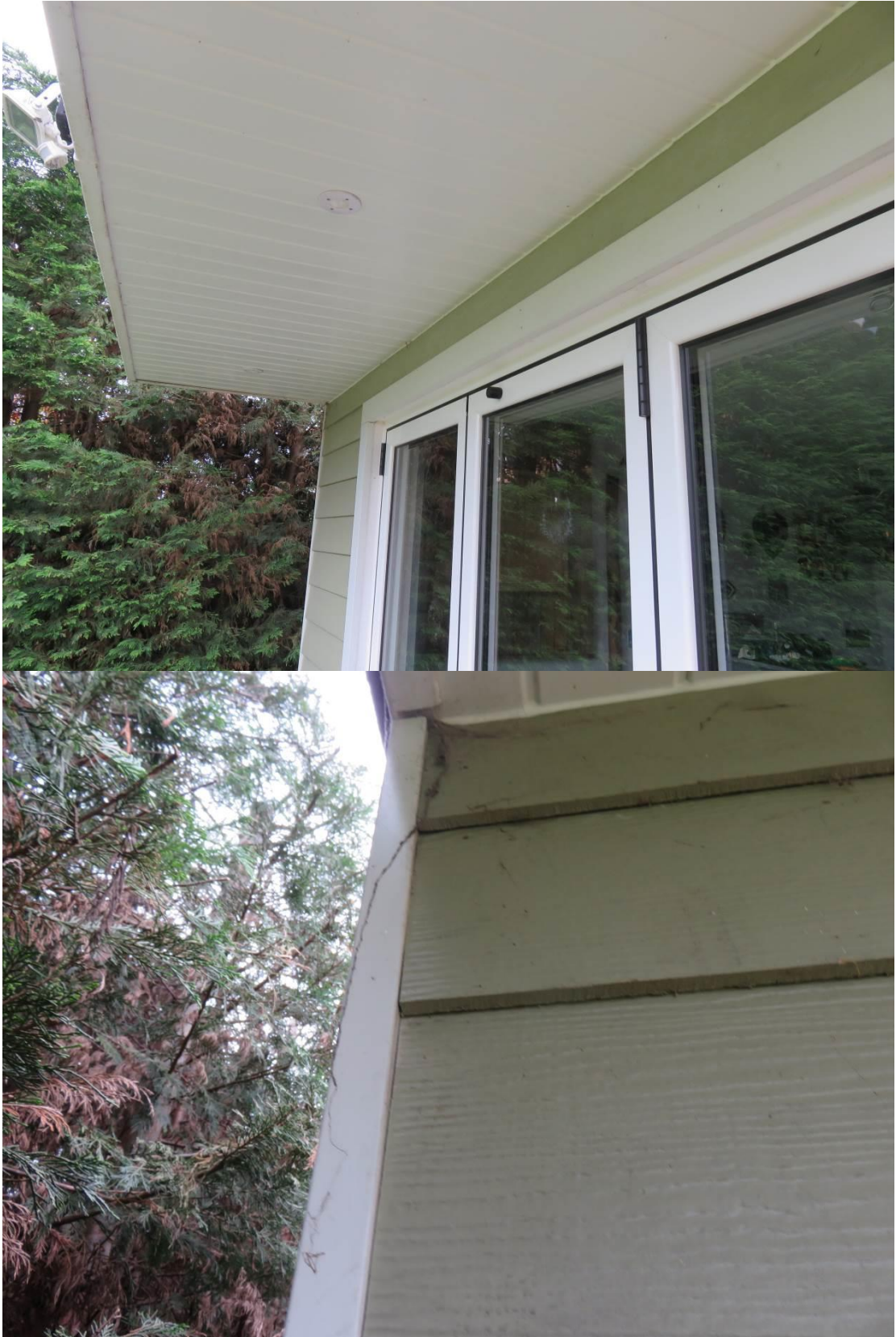
Photo 14/15 Felt Roof and cladding construction, No evidence recorded.
