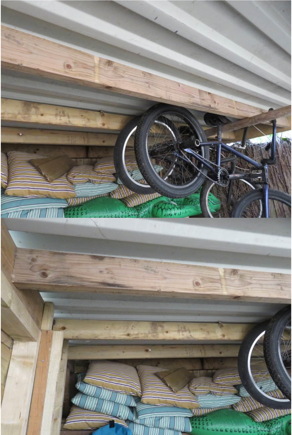
Photo 10/11 Open porch construction, No evidence recorded.
