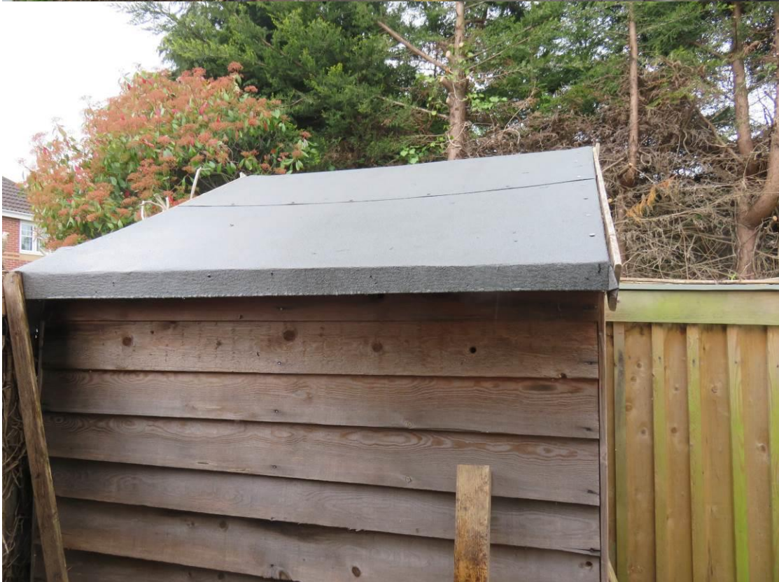
Photo 8/9 Out building with single skin construction with no/very limited crevice opportunity. Felt overlap cobwebbed with no crevice behind as single sheet roof construction. No evidence recorded.
