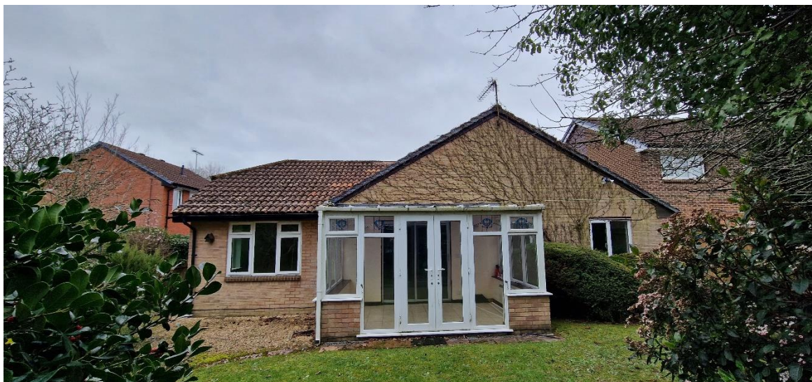
Picture 2: Showing the rear elevation.
