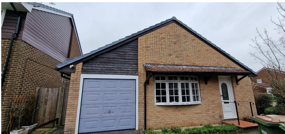
Picture 1: Showing the front elevation showing the weather boarding above the garage door.
