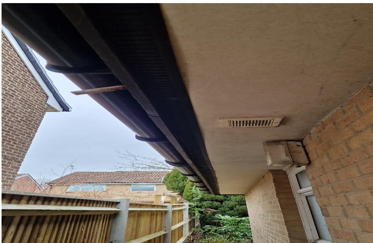
Picture 5: Showing the eaves and soffits.
