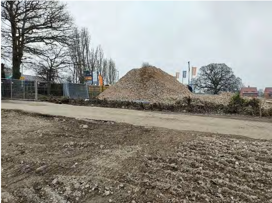
Plate 7 – View south of the crushed demolition material stockpile and hardstanding in the east of the site
