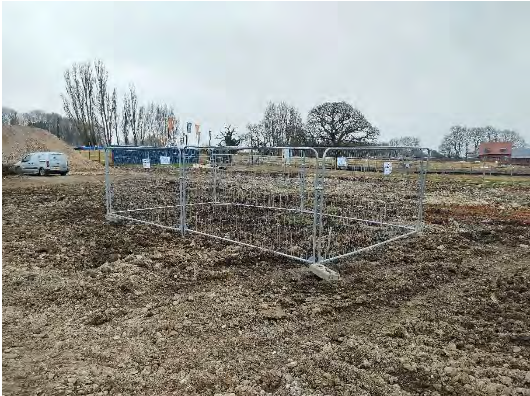
Plate 5 – Area of soft ground in the centre of the site
