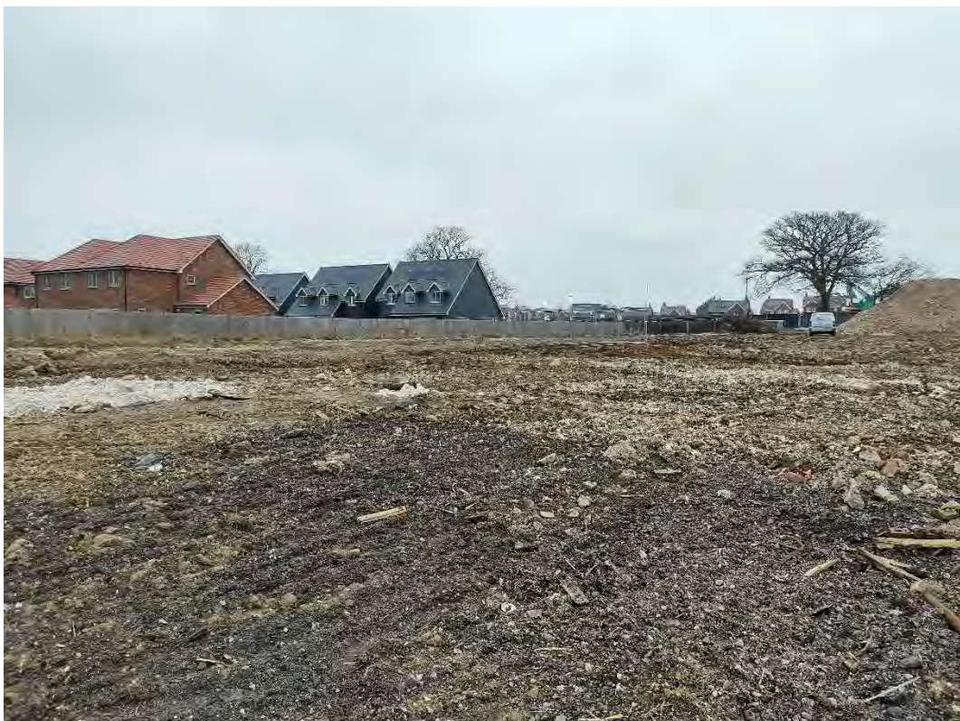
Plate 2 – View northeast across the site
