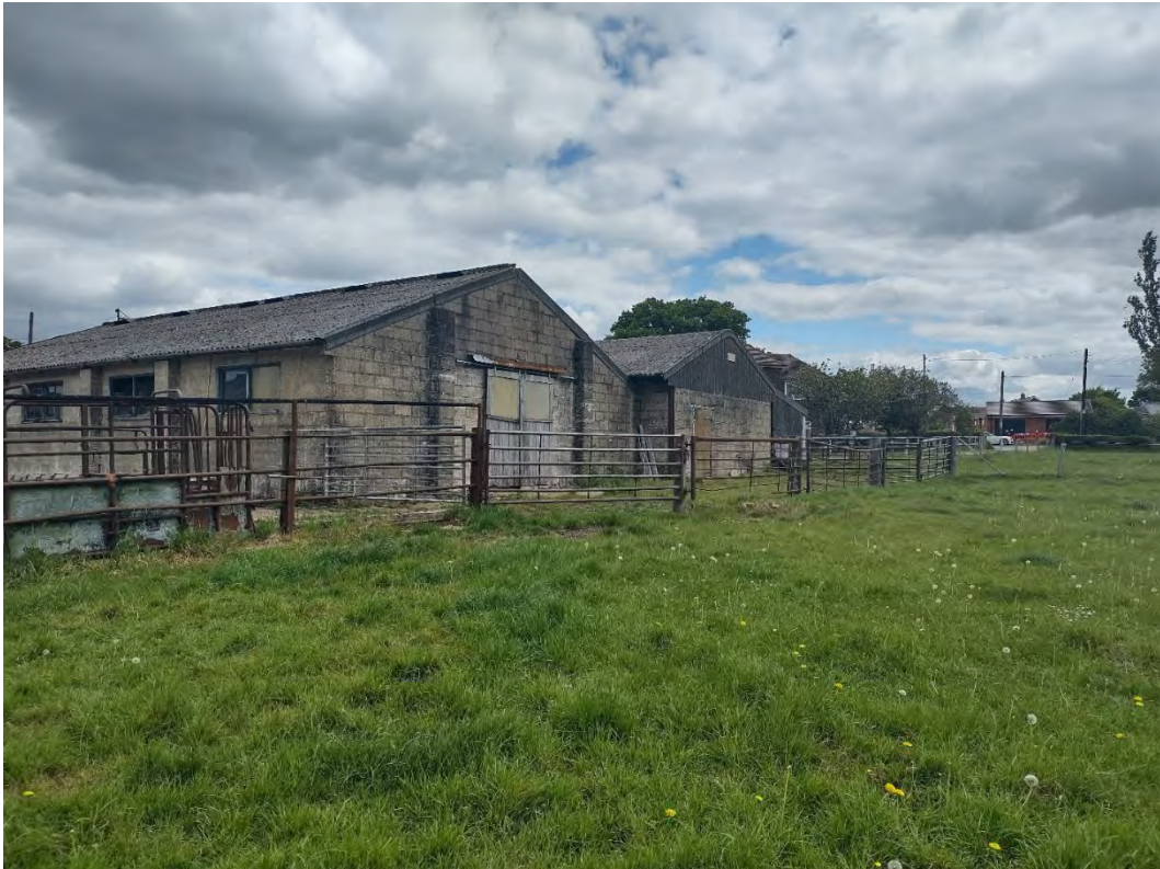
Plate 7 – View northeast across the site
