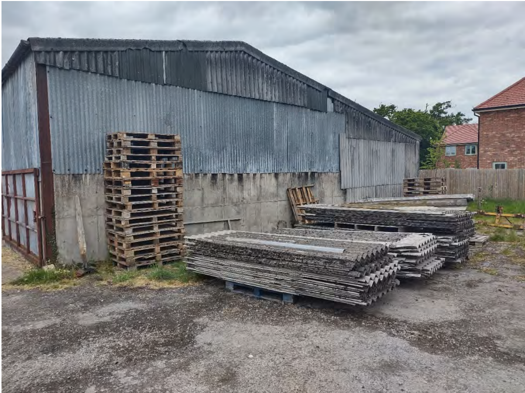
Plate 17 – Stacks of asbestos cement east of the northernmost barn
