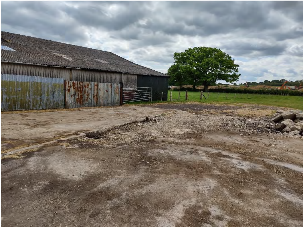
Plate 5 – View northeast across the site
