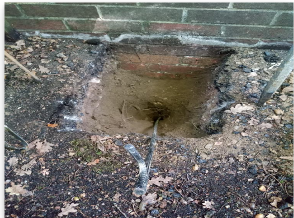
Fig 1.2: Trial Hole 1 Footing
