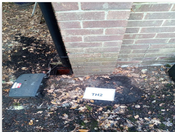
Fig 2.1: Trial Hole 2 Location
