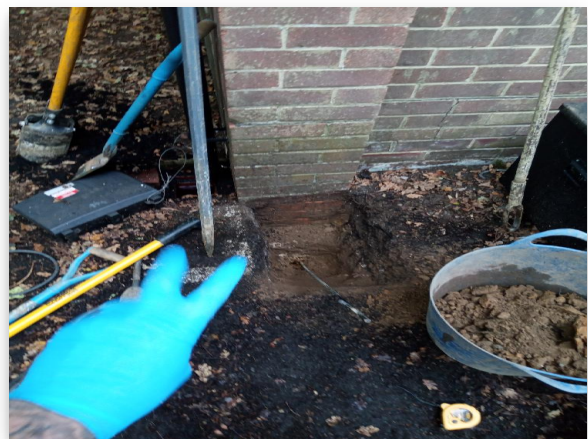
Fig 2.2: Trial Hole 2 Footing
