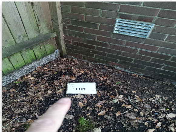
Fig 1.1: Trial Hole 1 Location
