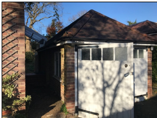
Figure 7 – south-eastern and south-western elevations of the garage with double doors
