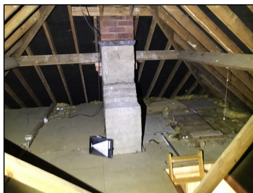
Figure 4 – roof void with boarded floor
