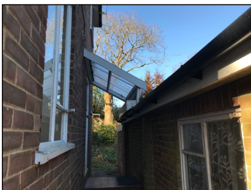
Figure 3 – lean-to roof on north-eastern elevation
