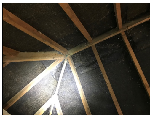
Figure 9 – internal view of the garage roof
