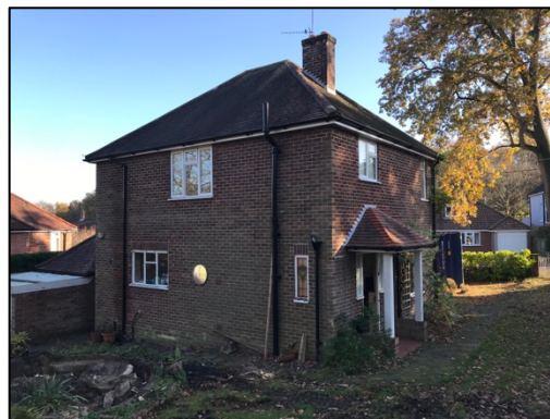
Figure 2 – south-western and north-western elevations of house with wooden framed porch
