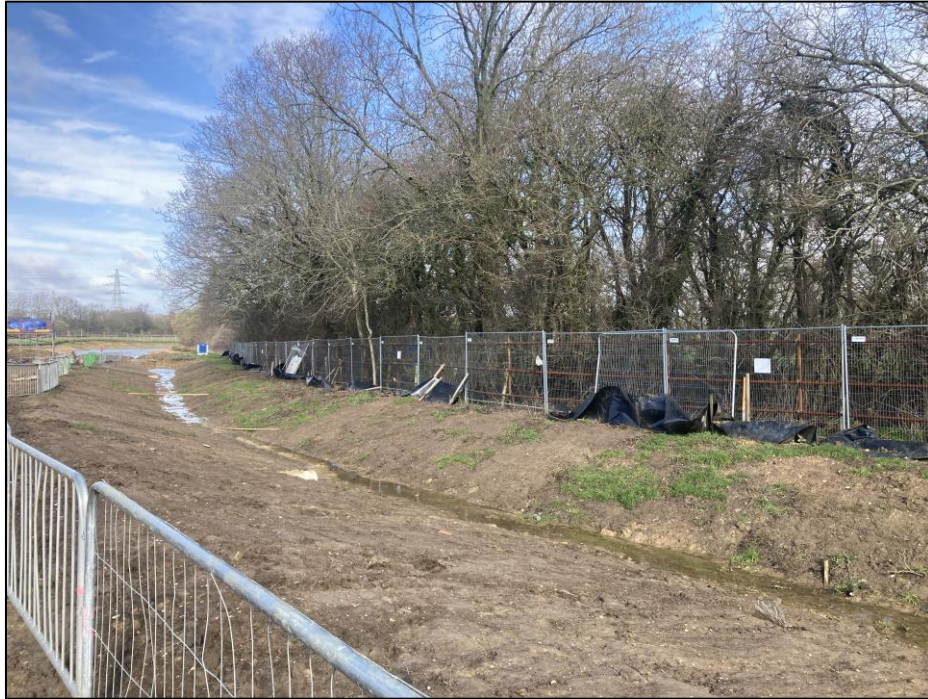
Figure 1: Photo Showing TPF around H8
