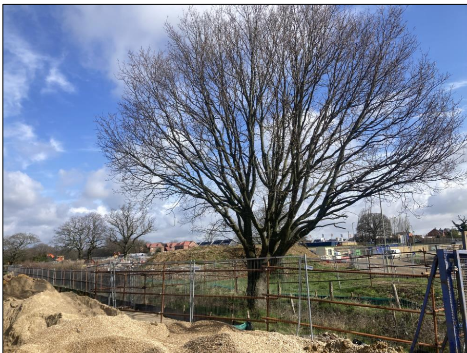
Figure 2: Photo Showing TPF around T7
