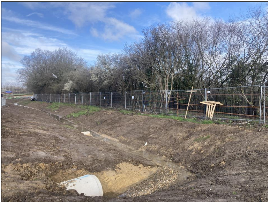
Figure 4: Photo Showing TPF around H8
