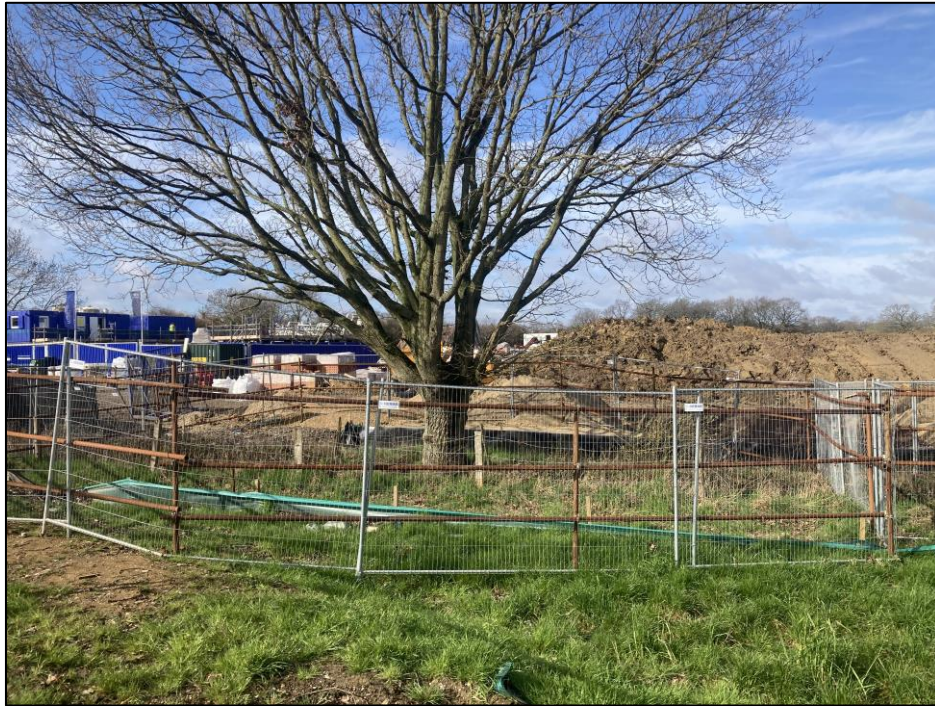
Figure 1: Photo Showing TPF around T7
