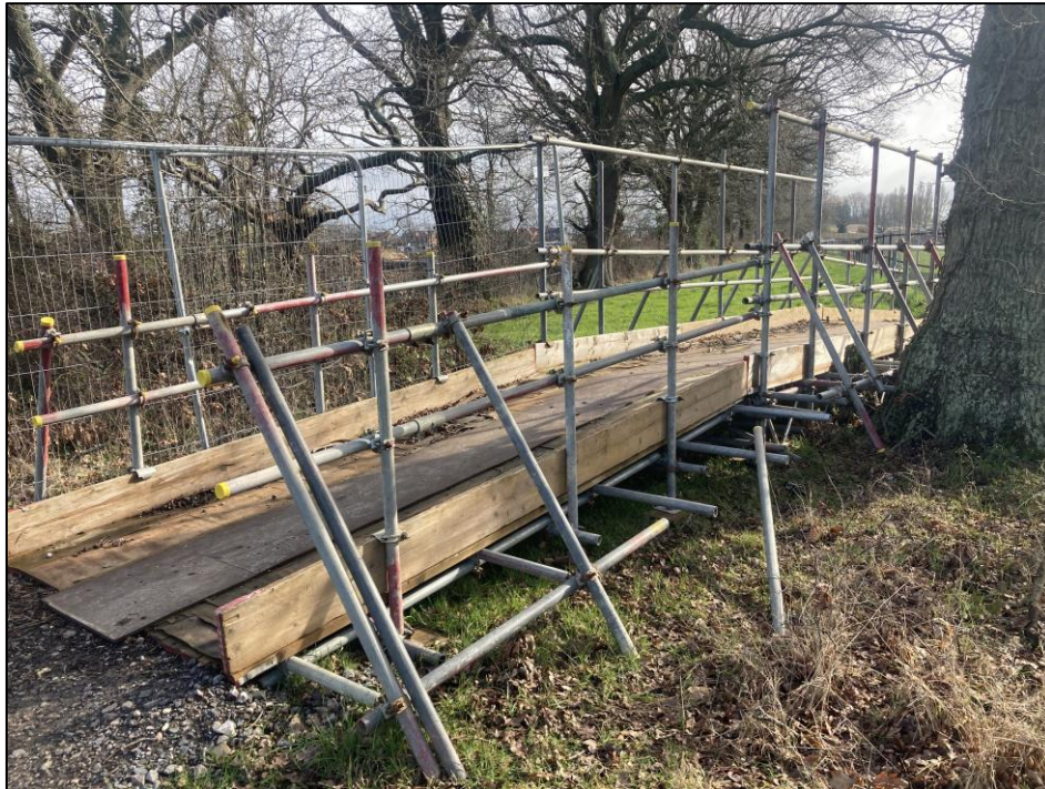
Figure 7: Photo Showing No-dig pedestrian bridge for the Public Right of Way through G12
