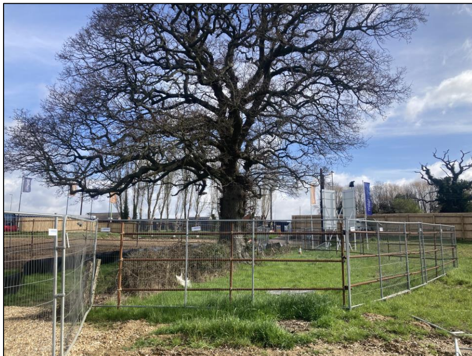
Figure 12: Photo Showing TPF around T19
