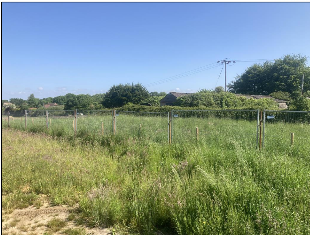
Figure 5 (above): Fencing erected to the West of H2
