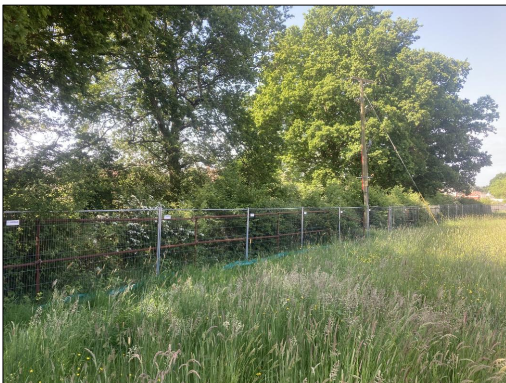
Figure 2 (below): Fencing erected to the North of H4, H6 and G8
