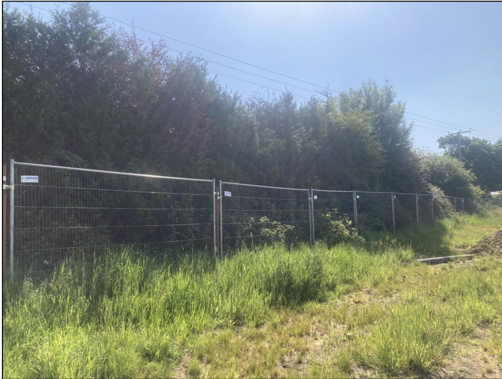
Figure 3 (above): Fencing erected to the West of boundary group H4 and H3
