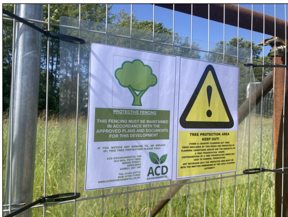
Figure 20 (below): Tree protection signage attached intermittently along fencing lines
