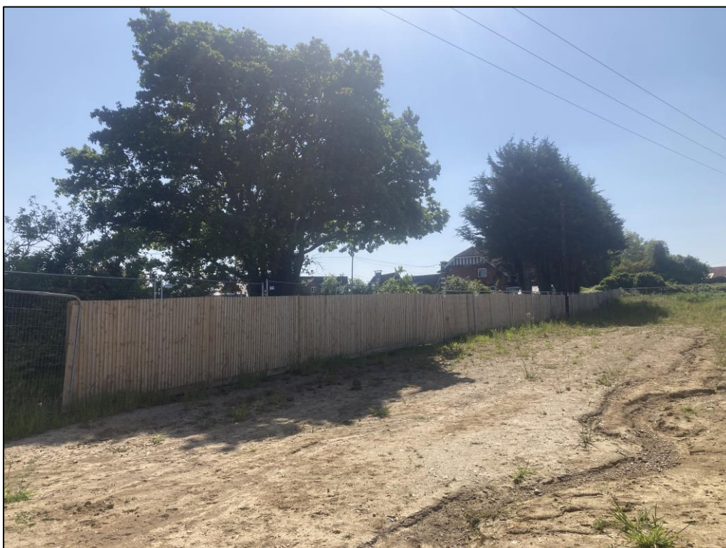
Figure 4 (below): Fencing erected to the West of H3 and G6
