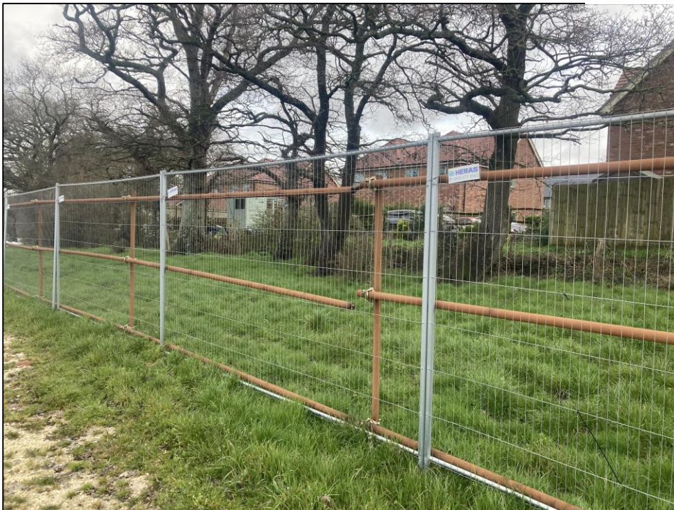
Figure 3: Photo Showing TPF erected to the West of G24 on the Eastern boundary of the site
