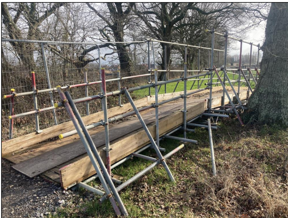
Figure 12: No-dig pedestrian bridge along the Public Right of Way that runs through the RPA of G12
