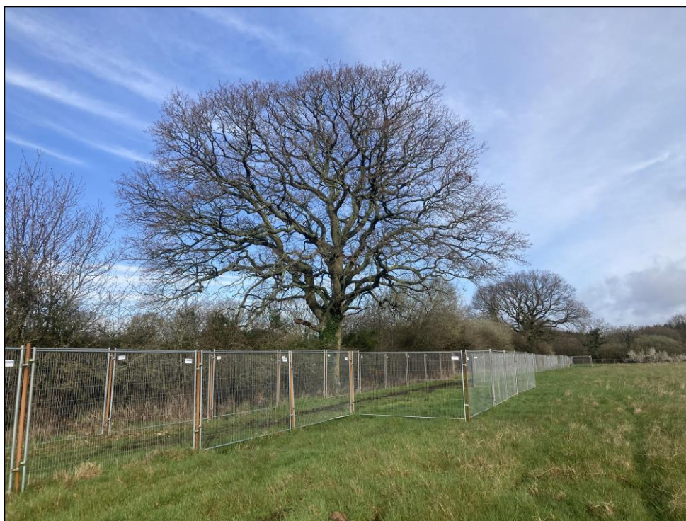
Figure 2: Photo showing tree protection fencing surrounding tree T15 & T16 - 'A' Category Oaks and T17 – 'B' category Oak
