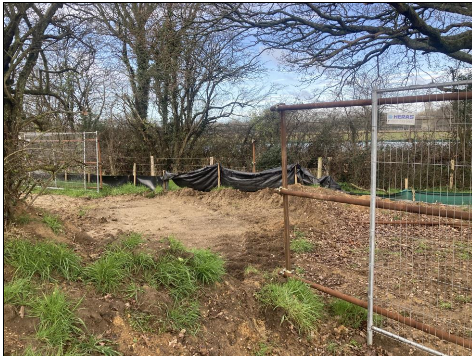
Figure 7: Section of missing fencing to the South of large Oak within G16
