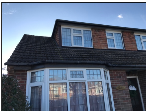
Figure 3 – north-eastern elevation with bay window and dormer windows
