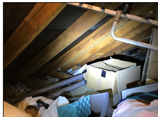
Figure 4 – roof void with bitumen lining and stored items
