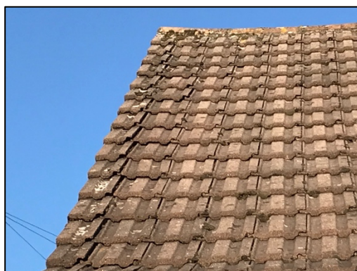
Figure 5 – lifted interlocking concrete tiles
