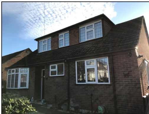
Figure 1 – north-eastern elevation and dormer windows
