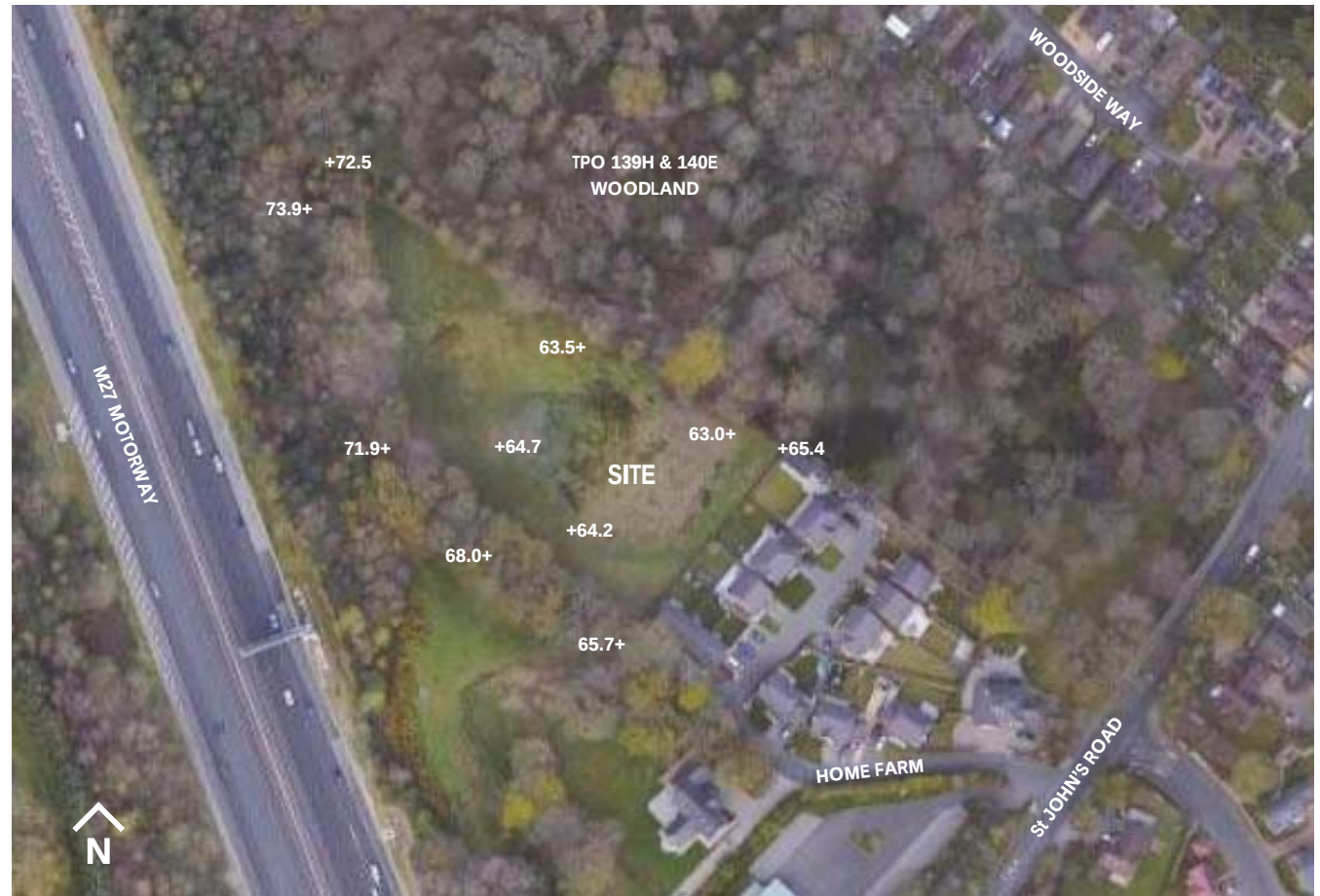
THE EXISTING SITE
