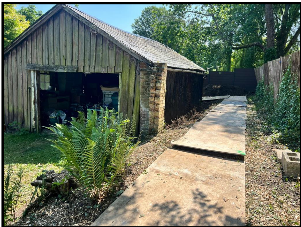
Plate 2: Ground protection.
