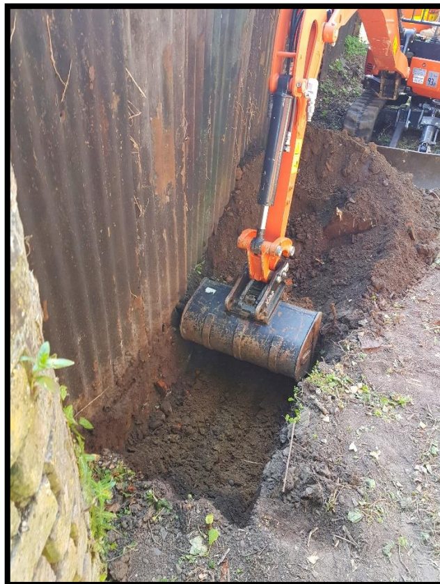
Plates 4: excavation of accumulated soil to top of foundations.
