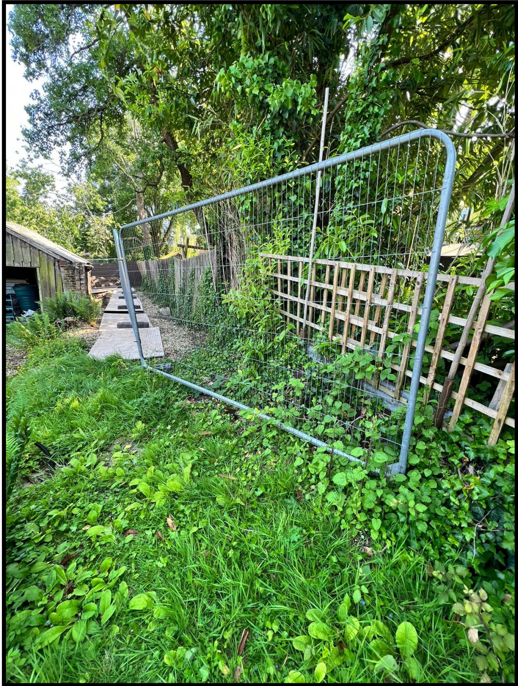
Plate 3: Tree protection installed.
