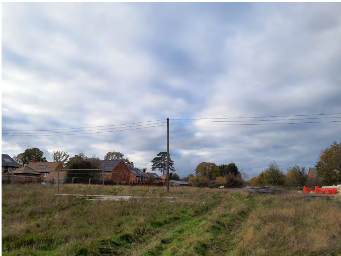
Plate 14: Overhead cables cross cutting the eastern soft landscaping.
