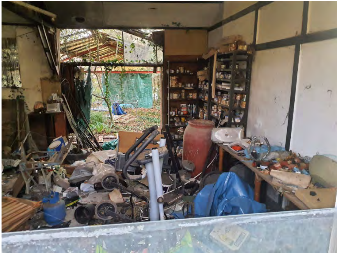
Plate 27: Paint cans in south-western workshop.
