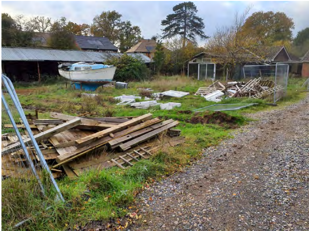
Plate 19: Stockpiles of wood and windows in the centre of the site.
