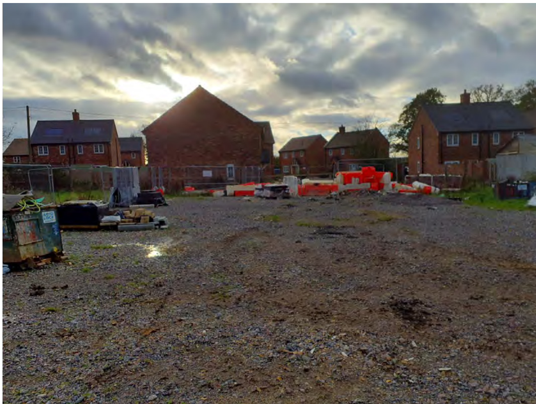
Plate 18: A small skip of materials and stockpiles of brick, sand and plastic bollards in the central portion of the site.
