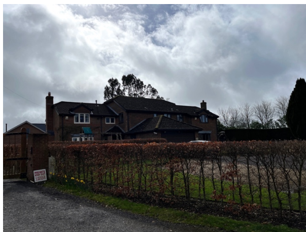
The barn-hipped roof of 'Corringham House'.
