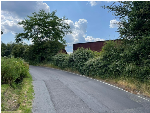
The application subject viewed from the northeast, on Grange Road.
