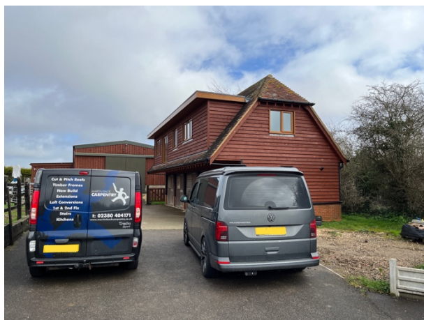
The existing building, viewed from the southwest.
