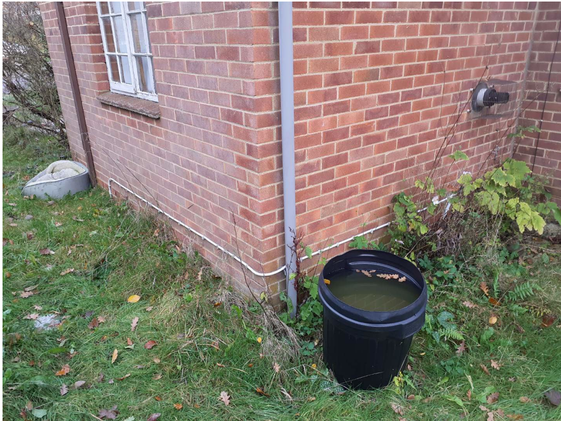
Plate 13: Potential buried service from the rear of the house.
