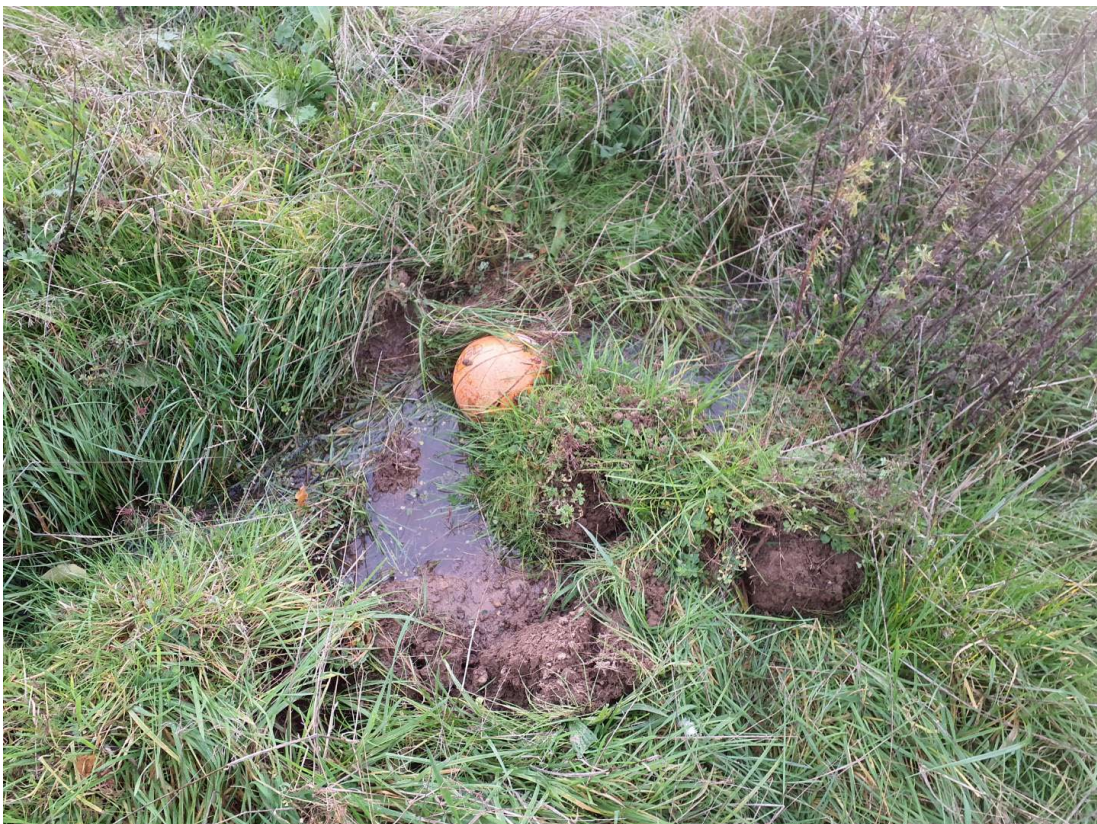
Plate 24: Evidence of high water table in the centre of the site.
