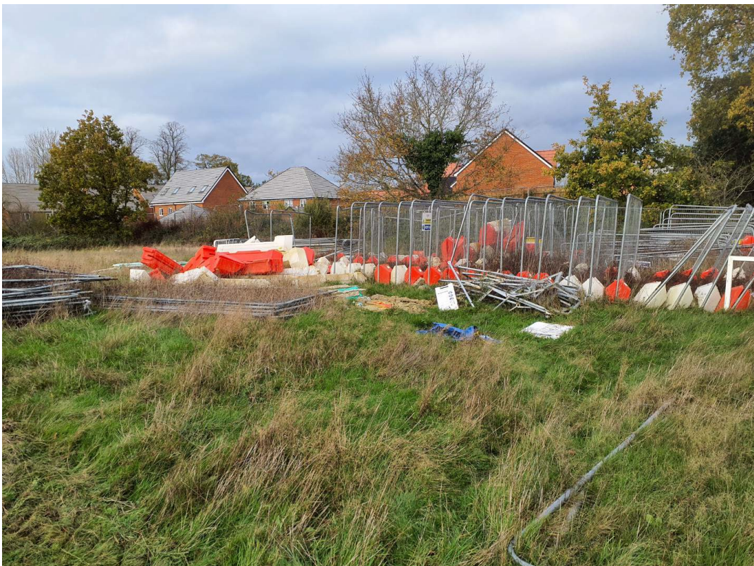
Plate 16: Stockpile of fencing in the centre of the eastern soft landscaping.
