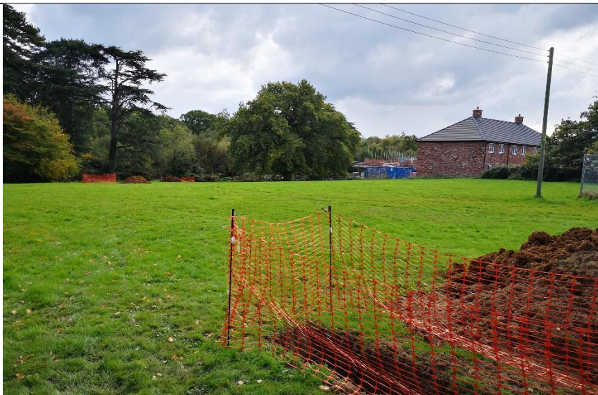
Photograph 8 Showing trial pitting in the south of the site area.
