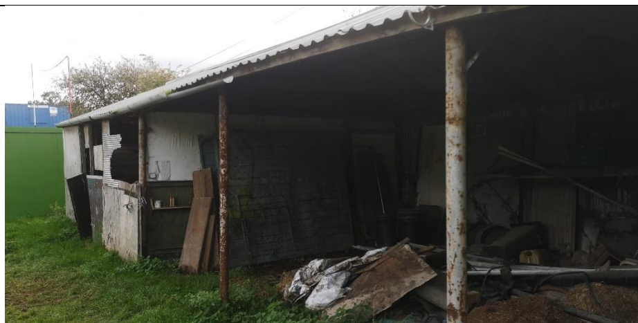
Photograph 4 Showing disused barn and stable to the west of the site area.
