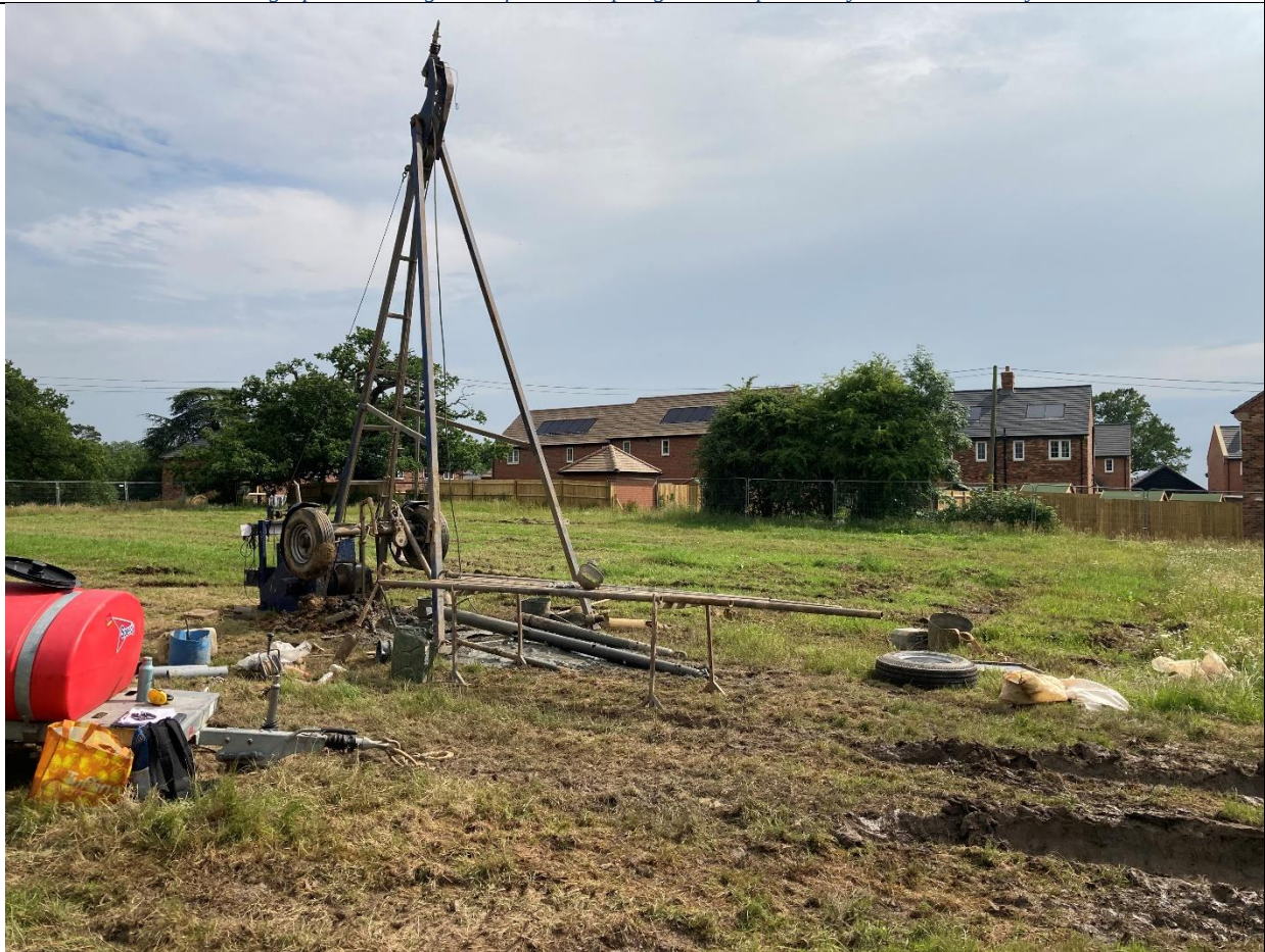
Photograph 4 Showing cable percussive borehole being advanced in the south of the site.
