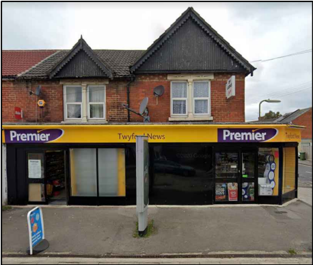
PHOTOGRAPH OF EXISTING ELEVATION A
