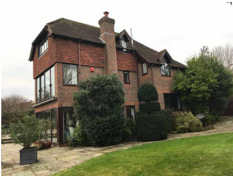
View of NE side elevation
