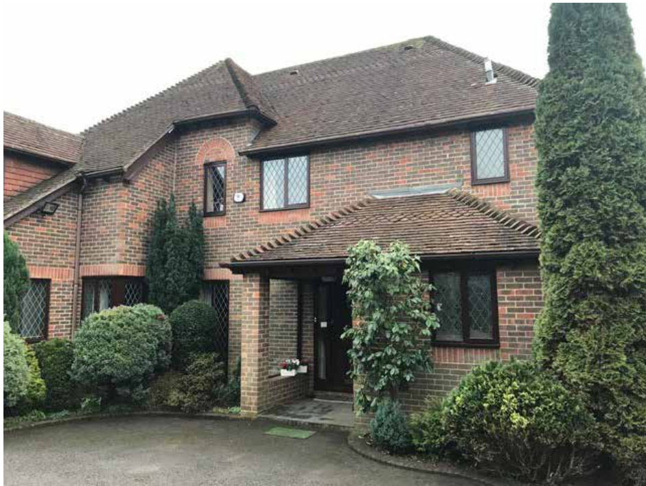
NW elevation looking towards the front porch, enlarged in 1995.
