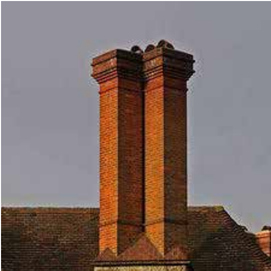
Brick detailing to chimneys
